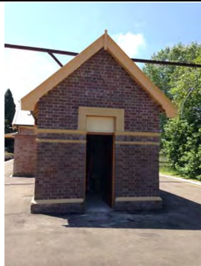
Photograph 4: Southern Storage Building Externals
