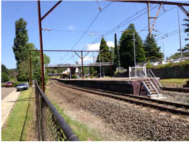
Photograph 1: Wentworth Falls Railway Station
