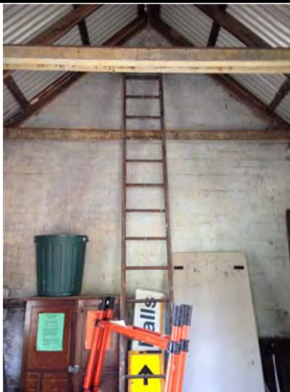
Photograph 5: Southern Storage Building Internals
