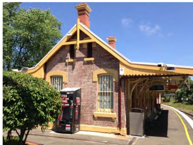
Photograph 6: Main Station Building
