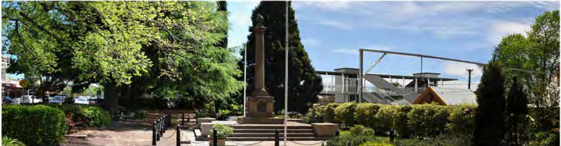
Photomontage PM 2 - View north to north east toward Wentworth Falls Station Proposal from Coronation Park
