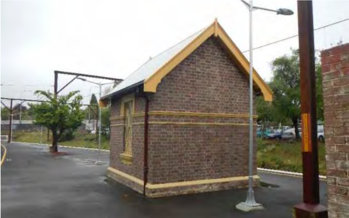
Image 10 Out of Shed building
