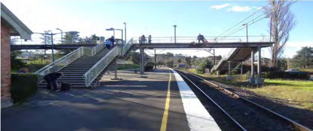
Image 2 View from platform looking north
