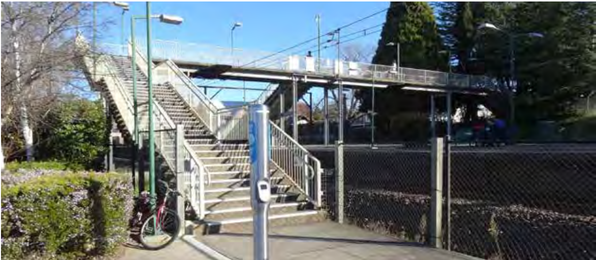
Image 3 View of stairs and footbridge on eastern side of station
