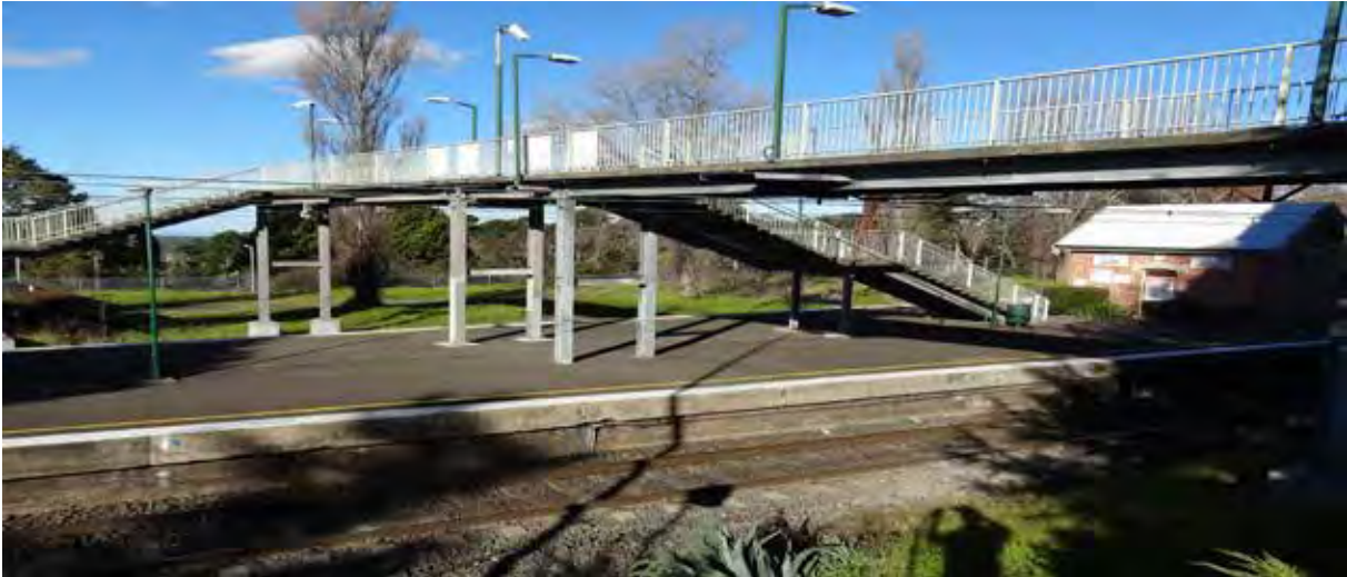
Image 1 View of existing footbridge looking south east
