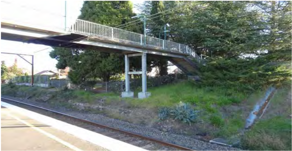
Image 4 View of Station Street stairs from station platform
