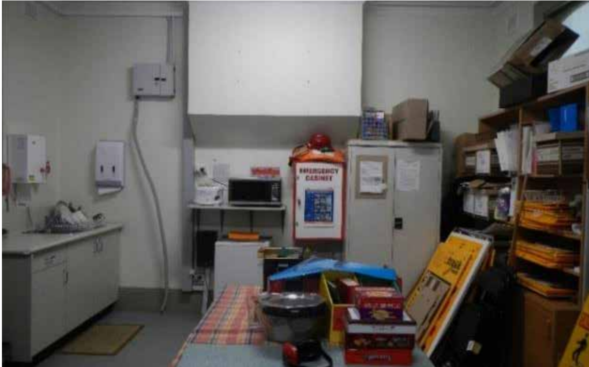
Image 7 Internal wall in current Station Manager's office proposed to be removed for larger waiting room
