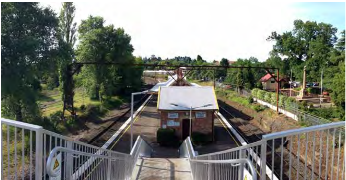
Image 5 View from footbridge looking south
