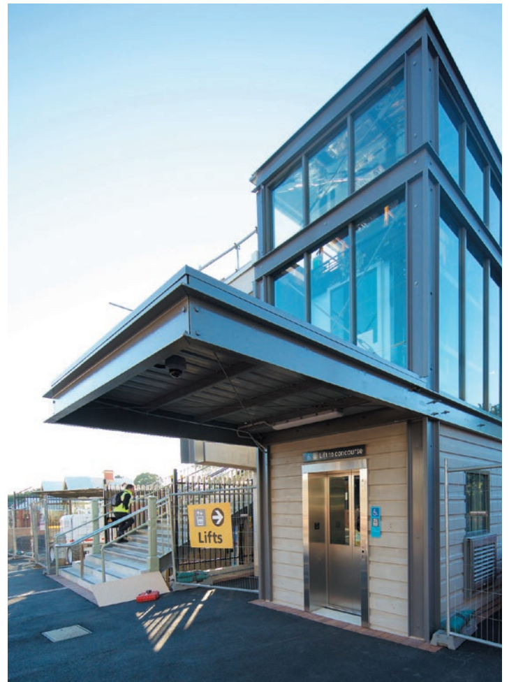
New lifts now available at Arncliffe Station
