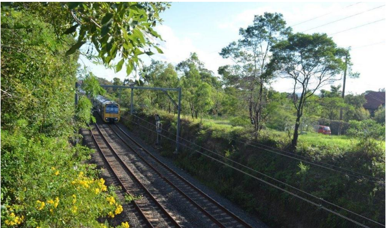
Figure 1.7 View of the proposed substation site looking east from Strickland Avenue
