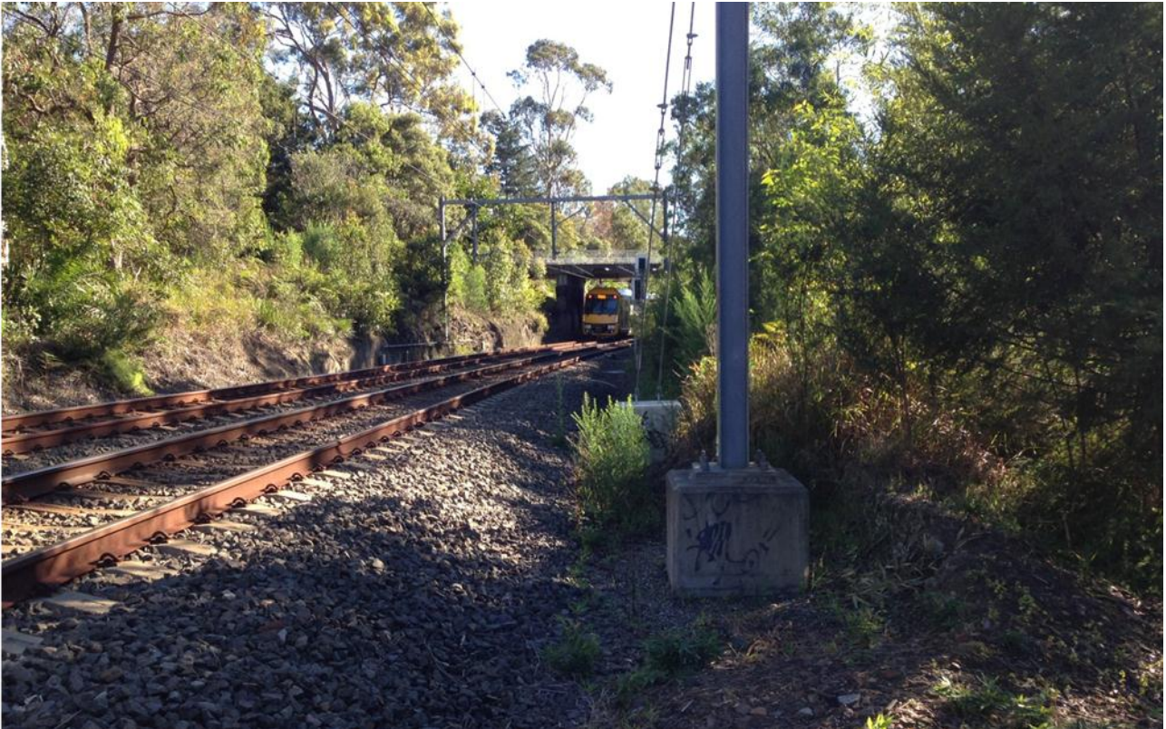
Figure 1.8 Typical example of the proposal site to the south of the substation site for the installation of the new combined services route, south of the Strickland Road Bridge
