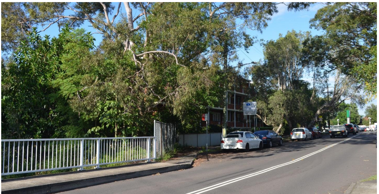
PHOTOGRAPH 5.2: RFB TO IMMEDIATE ON SOUTHERN SIDE OF STRICKLAND AVENUE (235-237 PACIFIC HIGHWAY)
