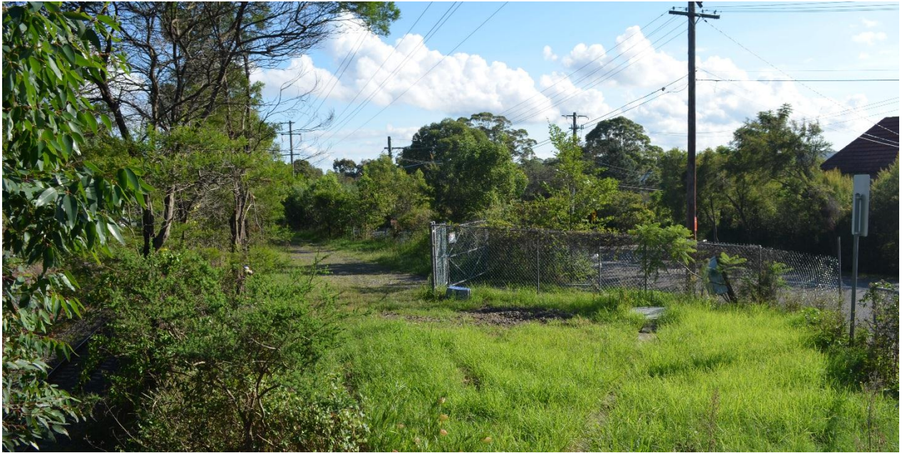
PHOTOGRAPH 2.1: VIEW OF SUBSTATION SITE LOOKING NORTH
