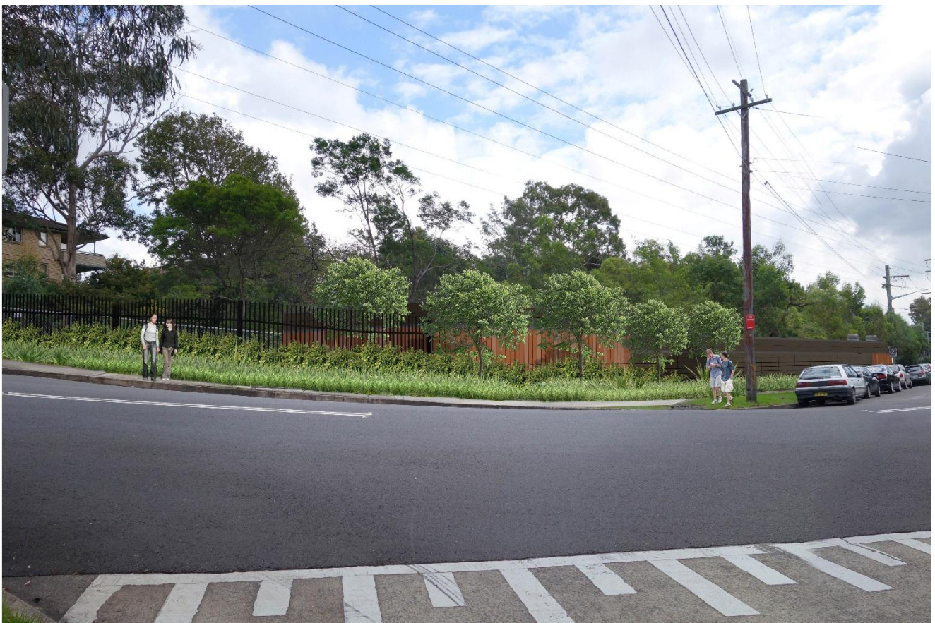
FIGURE 5.3: PHOTOMONTAGE B - PREDICTED VIEW OF SUBSTATION FROM CORNER OF STRICKLAND & LINDFIELD AVENUES
