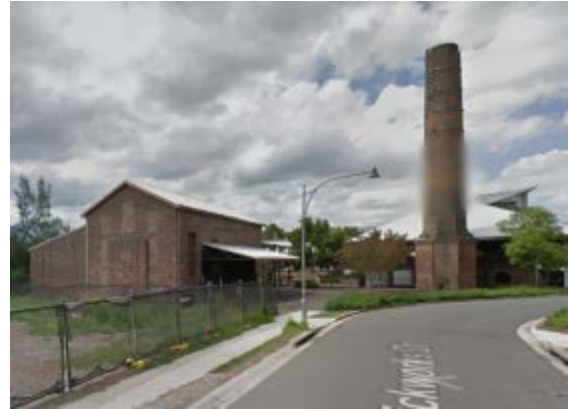
Figure 29: View of chimney and brickmaking plant facing north (Source: Google Maps)
