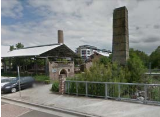
Figure 28: View of the chimney and kiln facing south (Source: Google Maps)
