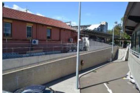
Figure 25: View of station building from existing car park facing south
