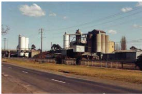
Figure 26: Photo of Millmaster Feeds Site in 1992 before demolition of buildings took place (Source: Holroyd City Council)
