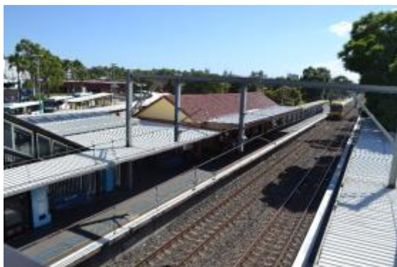
Figure 24: View of station building from overbridge facing north
