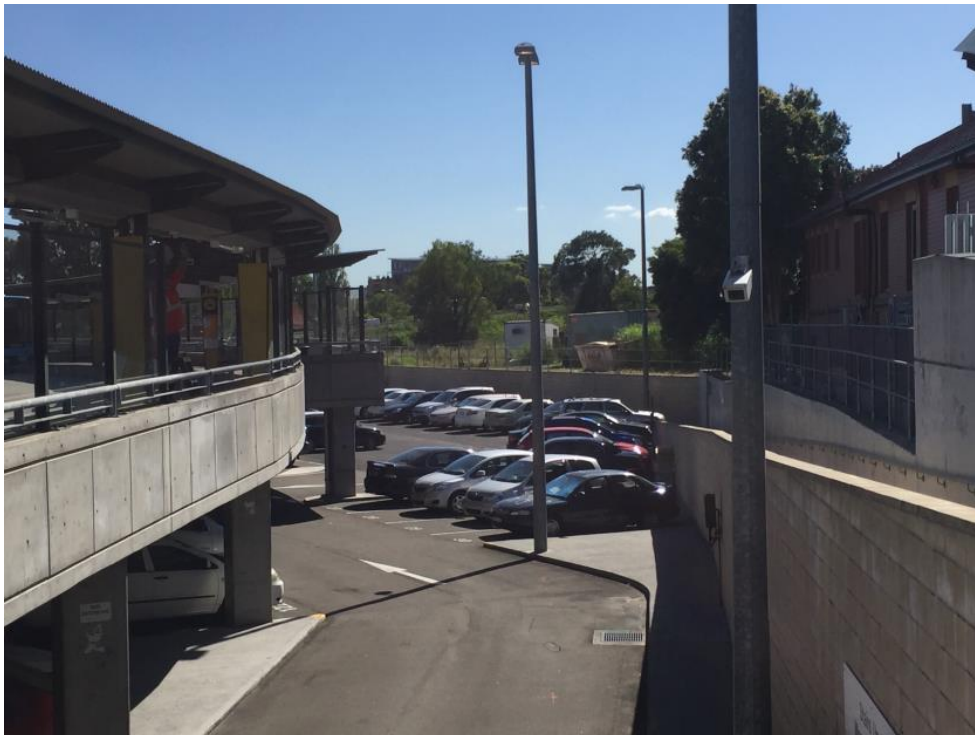
Figure 5 View of the existing lower ground car park (Site 1) from the station plaza looking north (bus interchange on the left)
