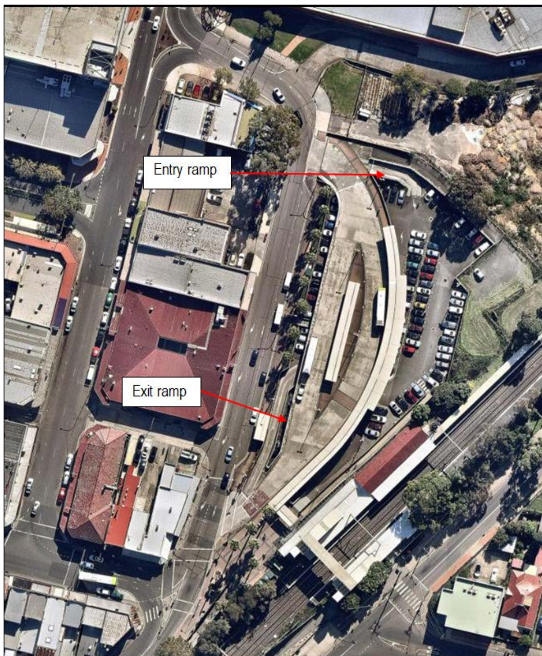
Figure 3-1 – Car park adjacent to train station and bus station, Merrylands
