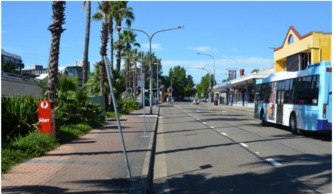
FIGURE 3-1: EXISTING BUS INTERCHANGE SEEN FROM TERMINAL PLACE
