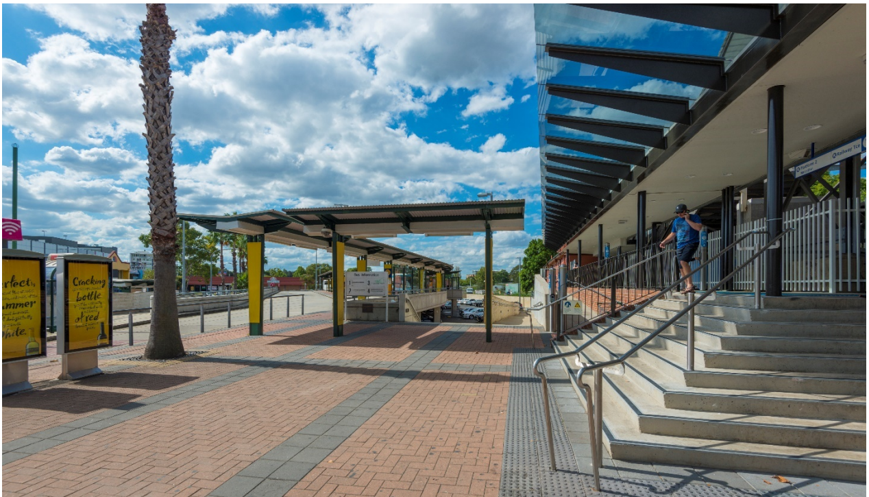
FIGURE 5-3: EXISTING VIEW FROM STATION FORECOURT
