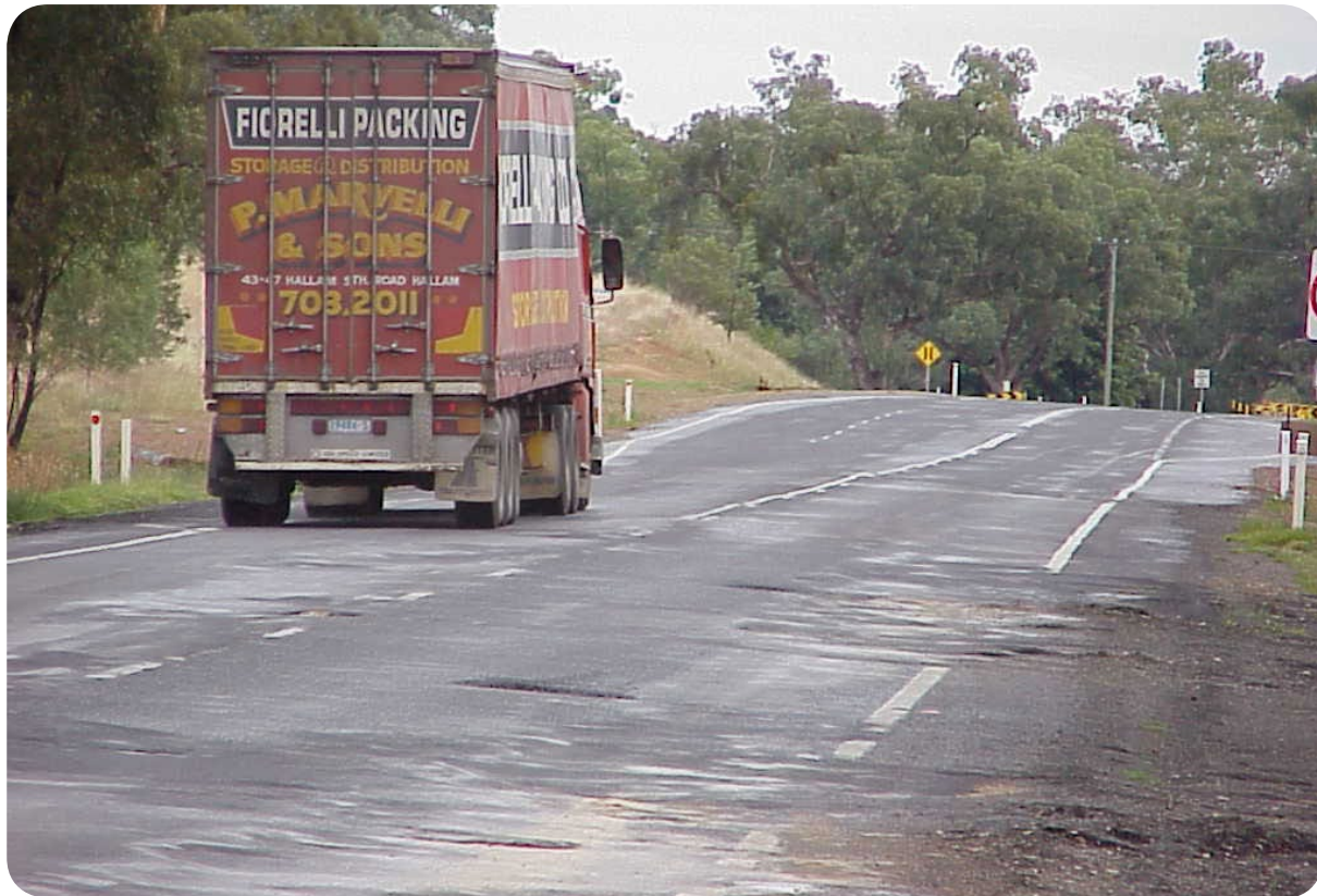
Pavement failures north of Forbes
