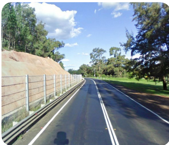
ARL 4 slope with rock bolting, shot-crete and rock fall fencing near Coonabarabran.
