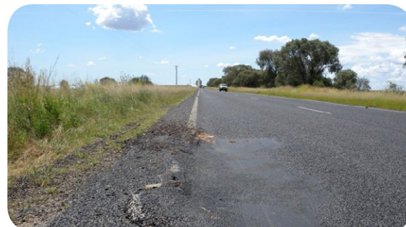
Typical edge pavement failure
