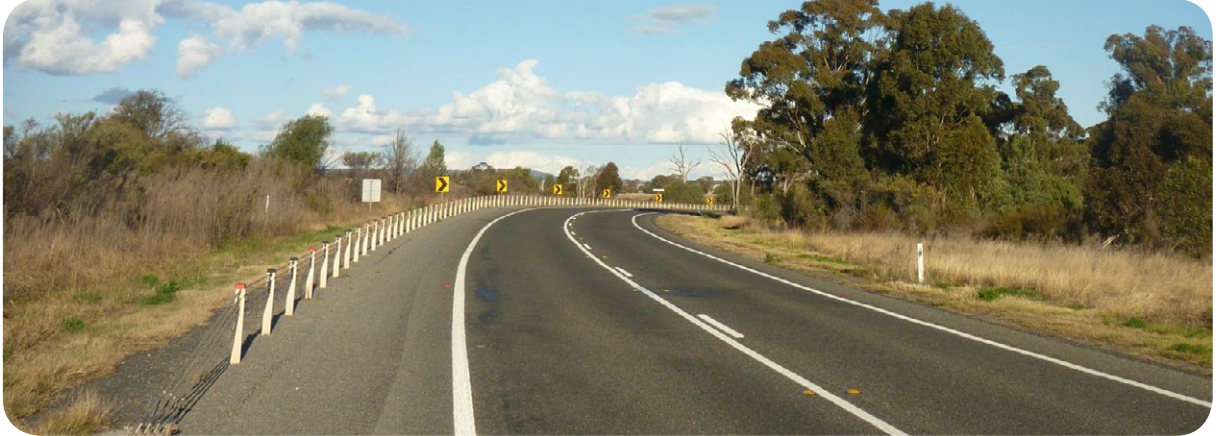
Wire rope safety barrier on road curve near Trewilga
