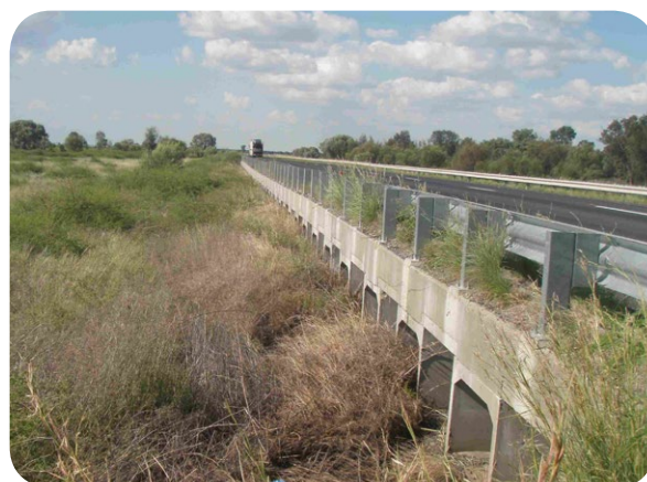
225 cell box culvert north of Moree
