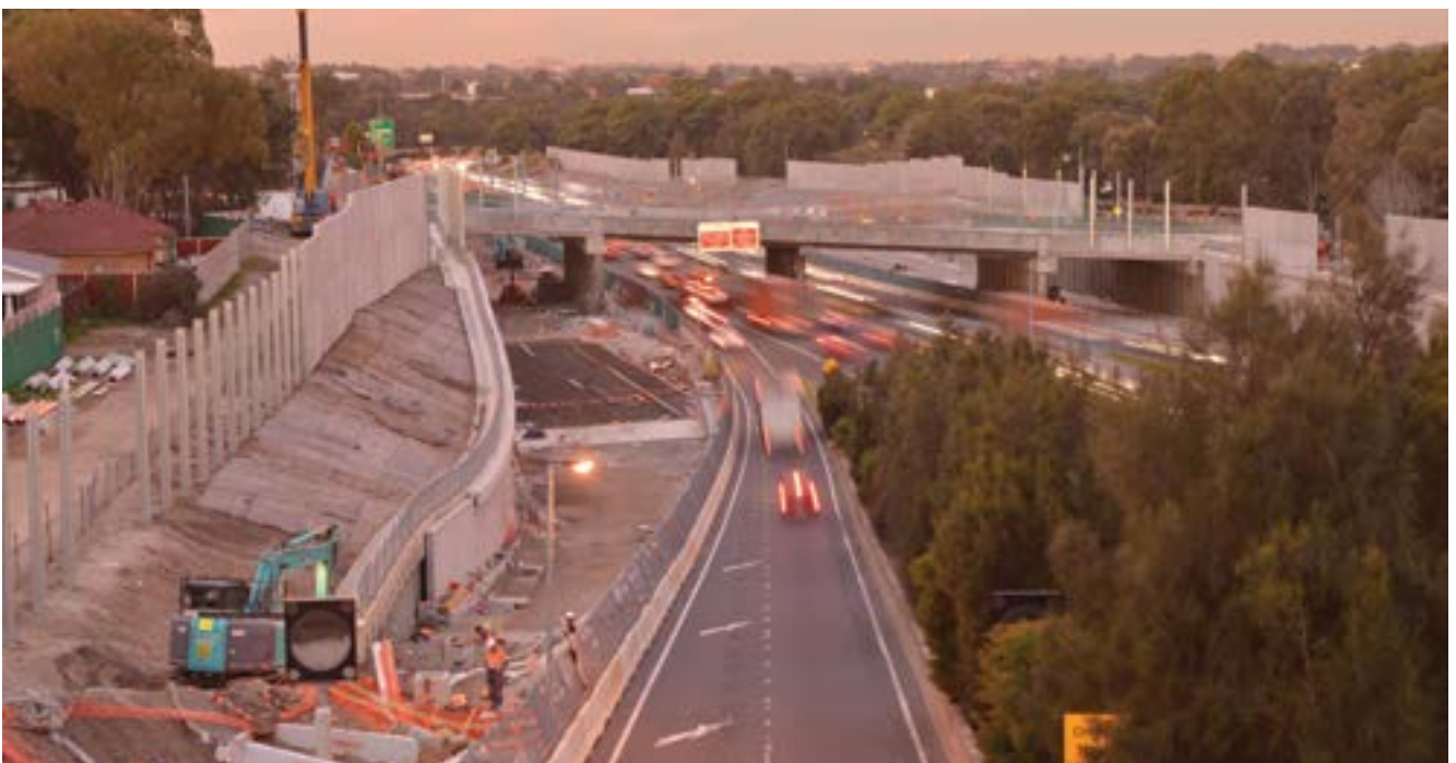
King Georges Road Interchange upgrade, Beverly Hills
