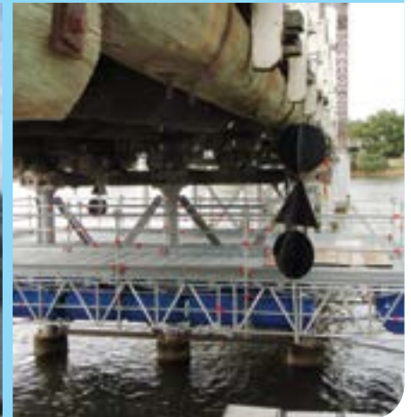
A suspended scaffold is floated into position for below deck works
