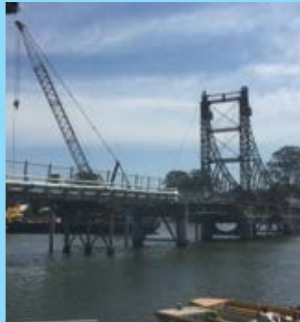
Restoration work underway
