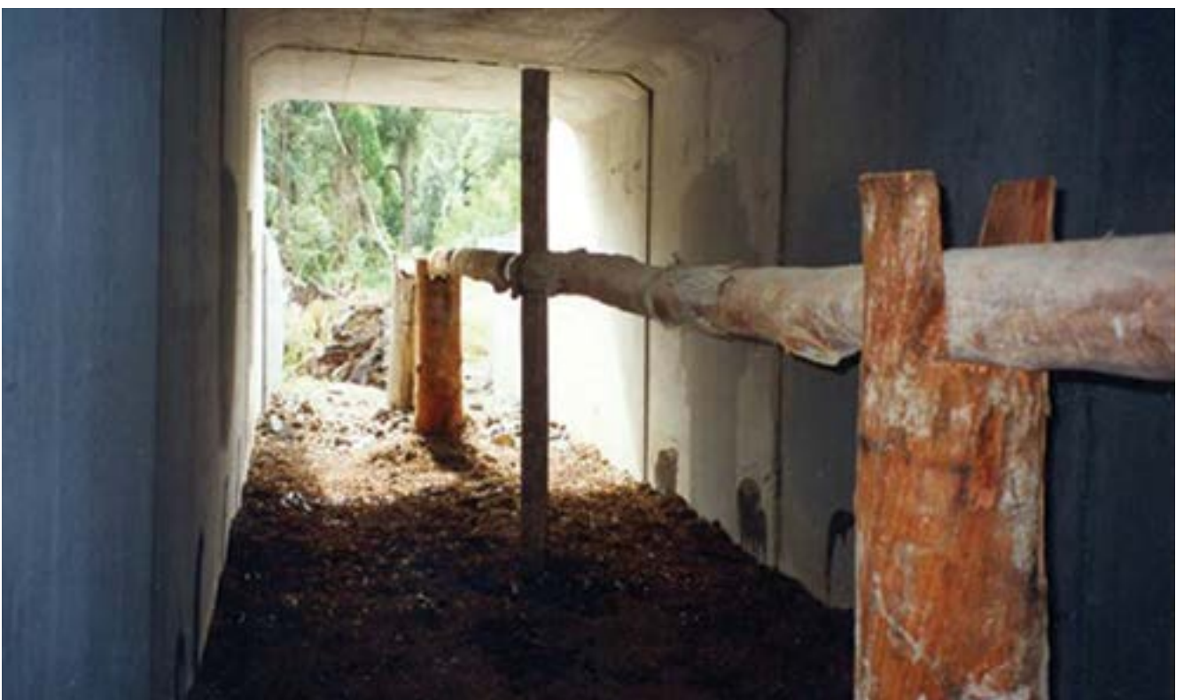
View through a recently constructed fauna underpass structure, Pacific Highway
