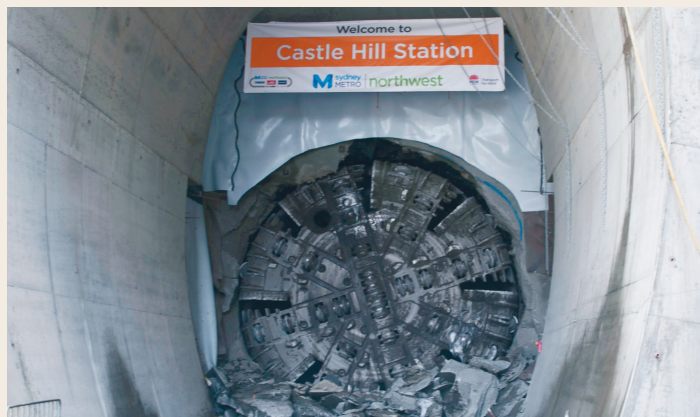
October 2015: Size and scale of a TBM in action at Castle Hill
