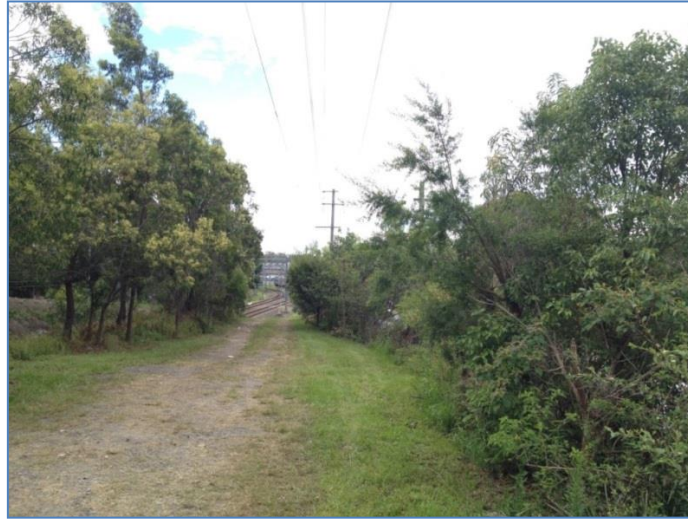
Figure 5: Views into the proposed Lindfield substation site. Artefact Heritage 2013.
