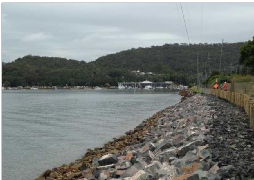
Example of a completed section of the rock armour wall at Brooklyn
