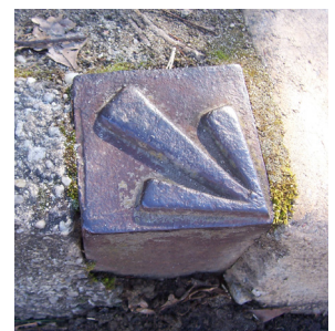
Alignment Pin references road alignment
