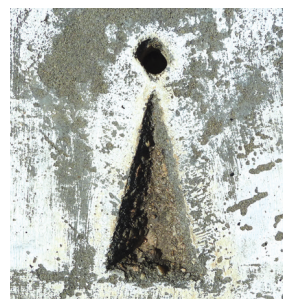
Drill Hole & Wing in Kerb references adjacent boundary corner
