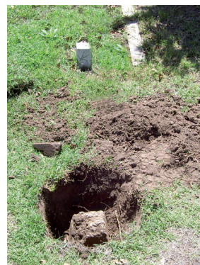
Concrete Block references boundary corner (peg)
