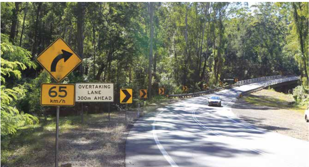
Photograph 1.5: Cabbage Tree Creek Bridge near Nelligen
