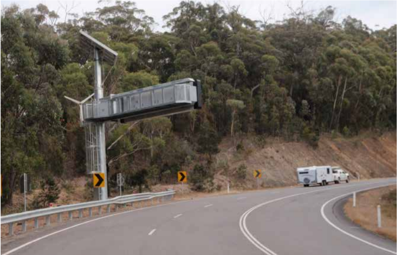
Photograph 2.13: Poorly located structure
