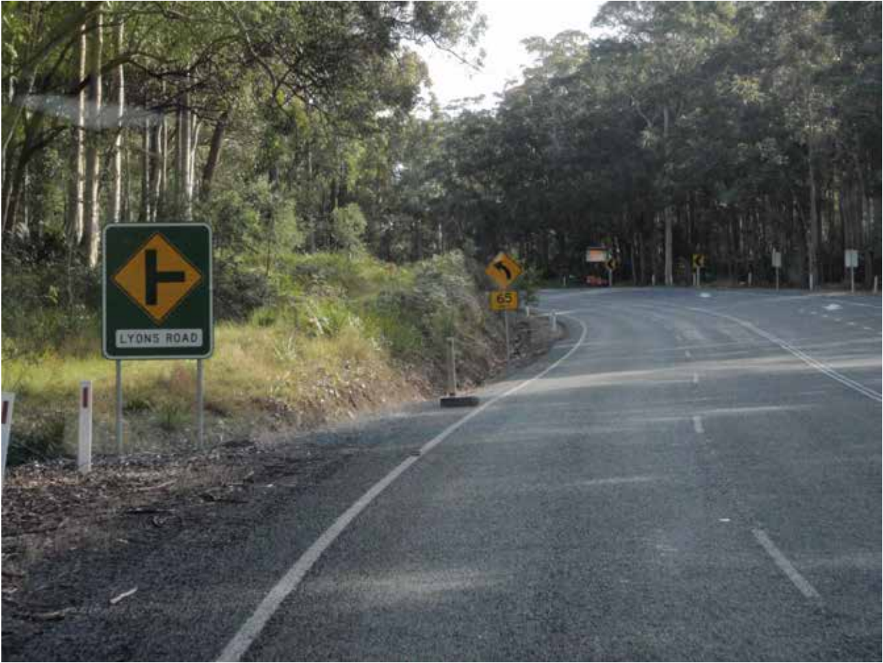
Photograph 2.5: Road junction in overtaking lane
