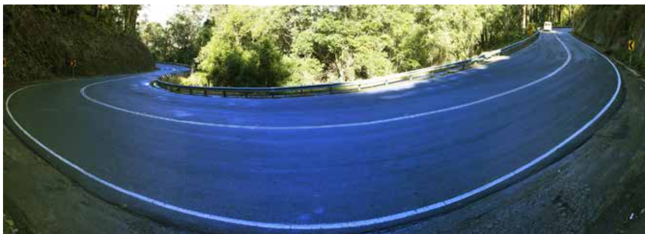
Photograph 2.4: Tight road alignment on the escarpment
