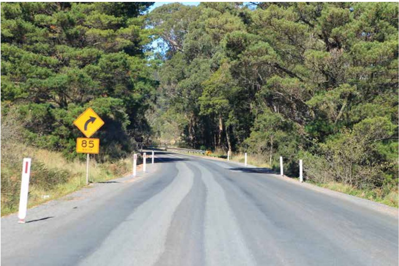
Photograph 2.9: Misleading curve warning sign
