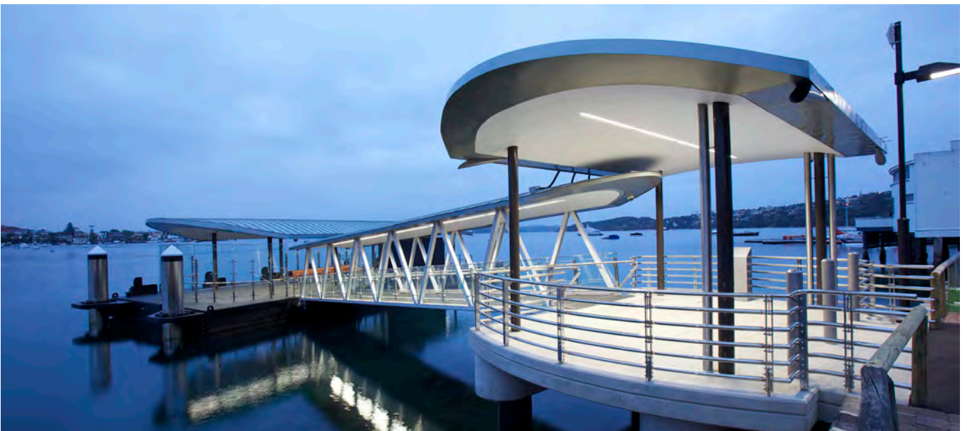
Lighting within wharf
