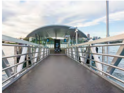
Open light steel truss system - gangway
