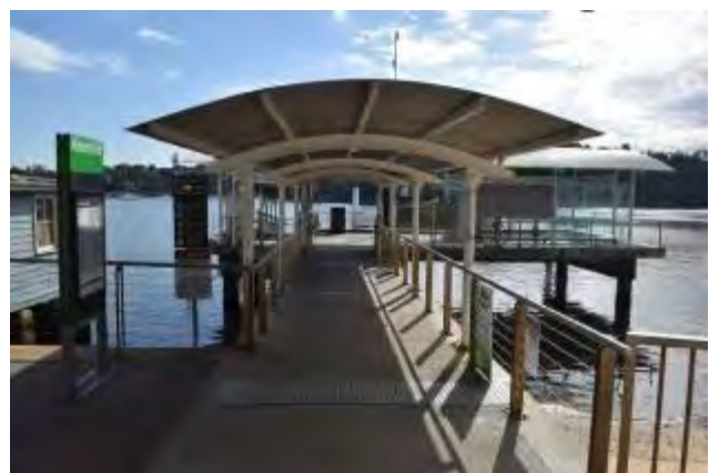
Figure 6: A view down the jetty towards the Parramatta River.
