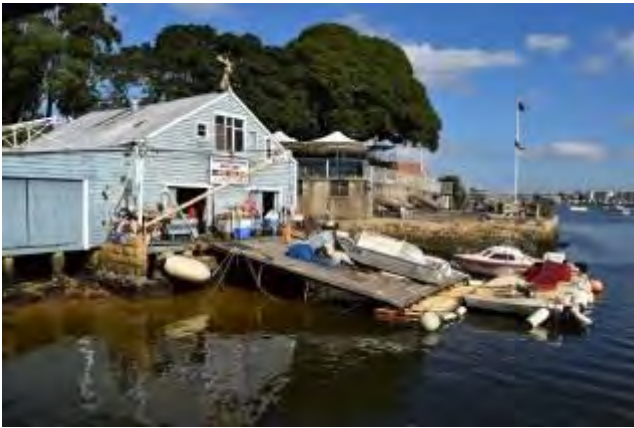
Figure 10: A general view of the northern façade of the Abbotsford Point Boatshed, facing the Paramatta River.
