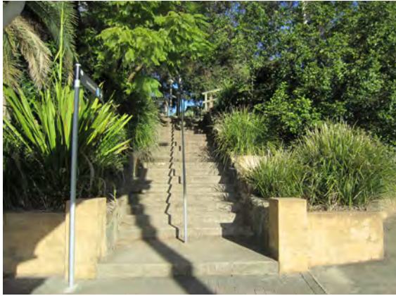
Existing steps and handrail
