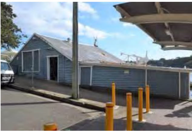
Figure 12: A general view of the southern façade of the Abbotsford Point Boatshed, on Great North Road. The historical sandstone kerbing is also visible here, in the foreground.
