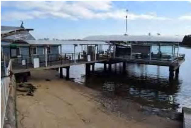
Figure 7: A view of the wharf in its entirety from the east.
