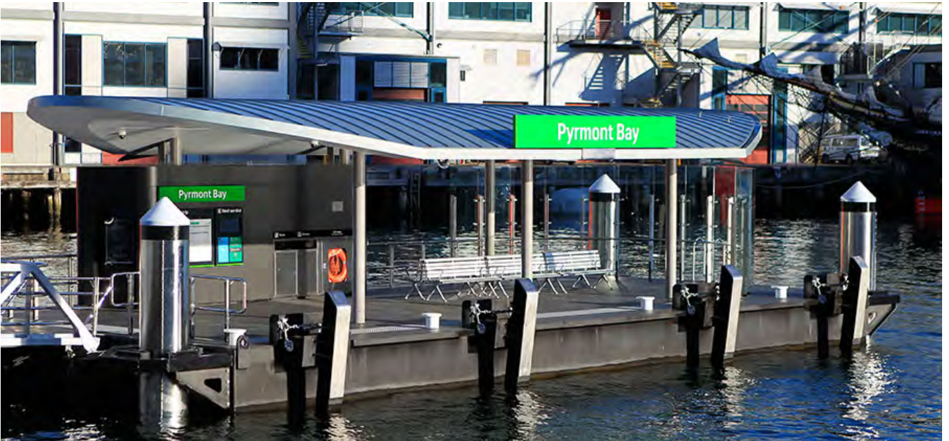
Pontoon with service pod
