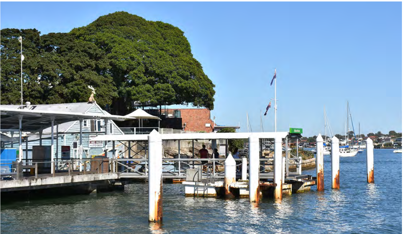
The existing wharf viewed from the water
