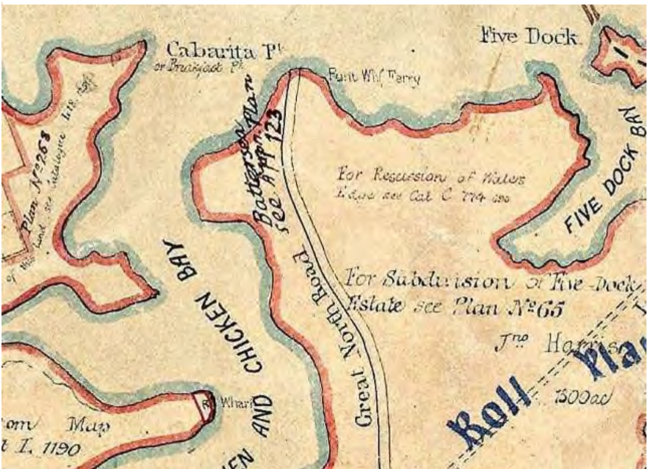
Figure 22: Excerpt of a parish map for Concord, undated, showing the existence of a 'Punt Wharf' at Abbotsford Point (circled in red). (Source: Lands & Property Information Historical Land Records Viewer)
