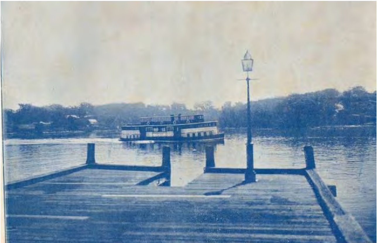
Figure 25: Abbotsford Wharf, with a view of a steam ferry, 1903. (Source: City of Canada Bay Council: Local Studies online archives. Originally from 'Abbotsford Park', a booklet published by Batt, Rodd & Purves Limited to promote an auction of land on 14 November 1903)
