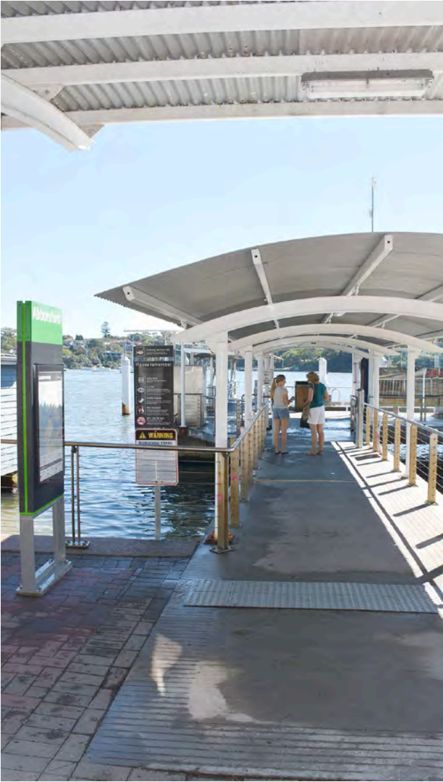
The existing Abbotsford wharf bridge
