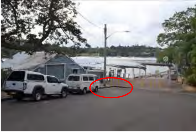
Figure 13: A view of the cul-de-sac of Great North Road, looking towards Abbotsford Wharf, with the sandstone kerbing indicated by the red ellipse.
