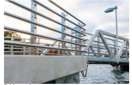
Bridge and gangway
