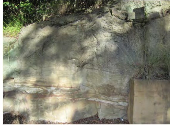
Sandstone of Werrell Reserve -pick marks in stone from early convict road construction
