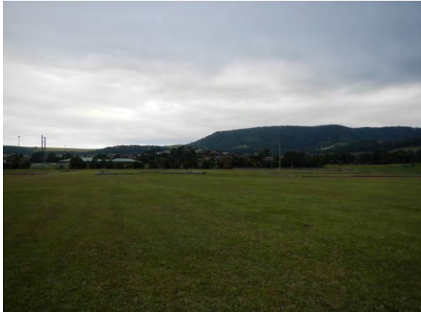
Plate 15: Survey Unit 4 – levelling and landscaping in pony club area, view to S.
