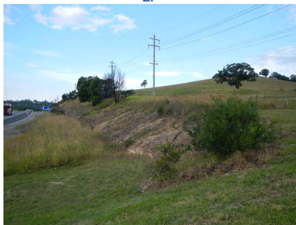
Plate 22: Survey Unit 6 – cutting through slope and crest landform to south of East West Link, view to E.
