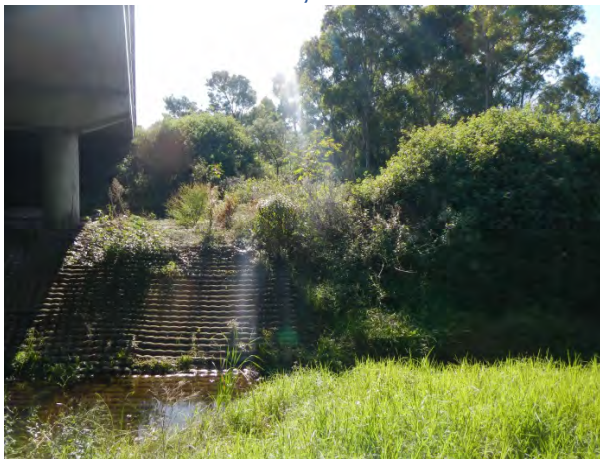
Plate 3: Survey Unit 1 – modifications made to Duck Creek, view to N.
