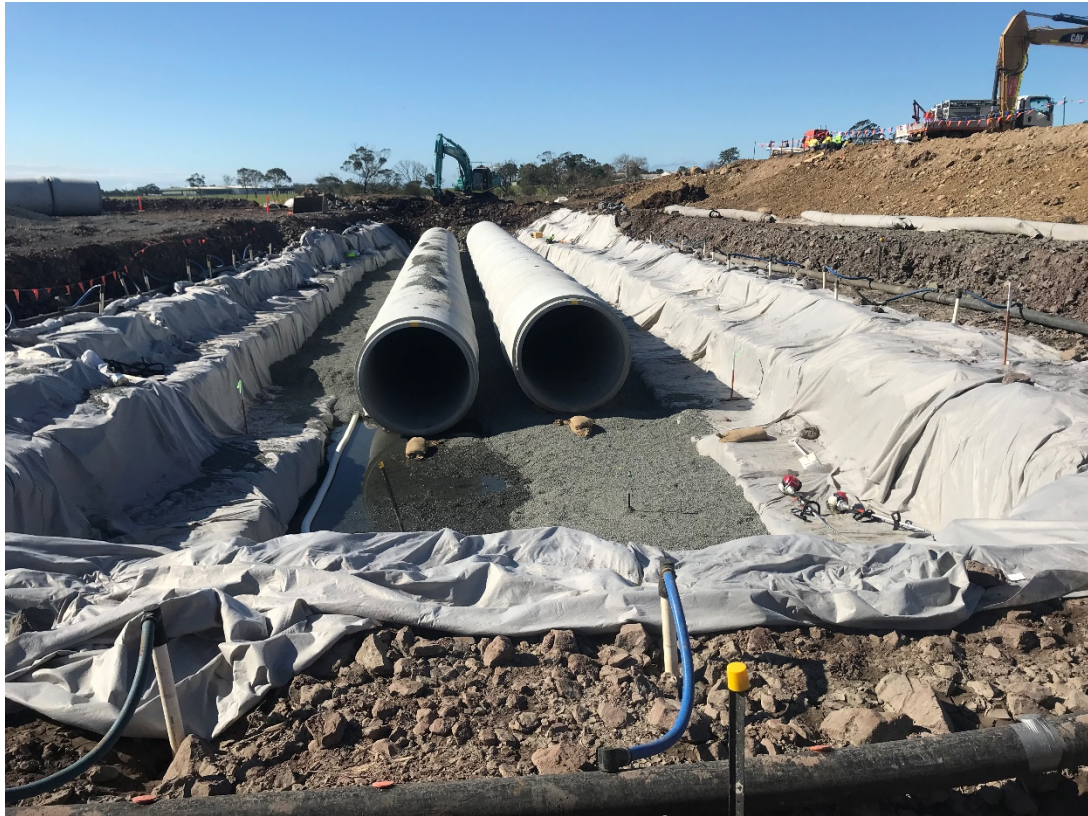
Figure 2-4: Early installation of transverse drainage
