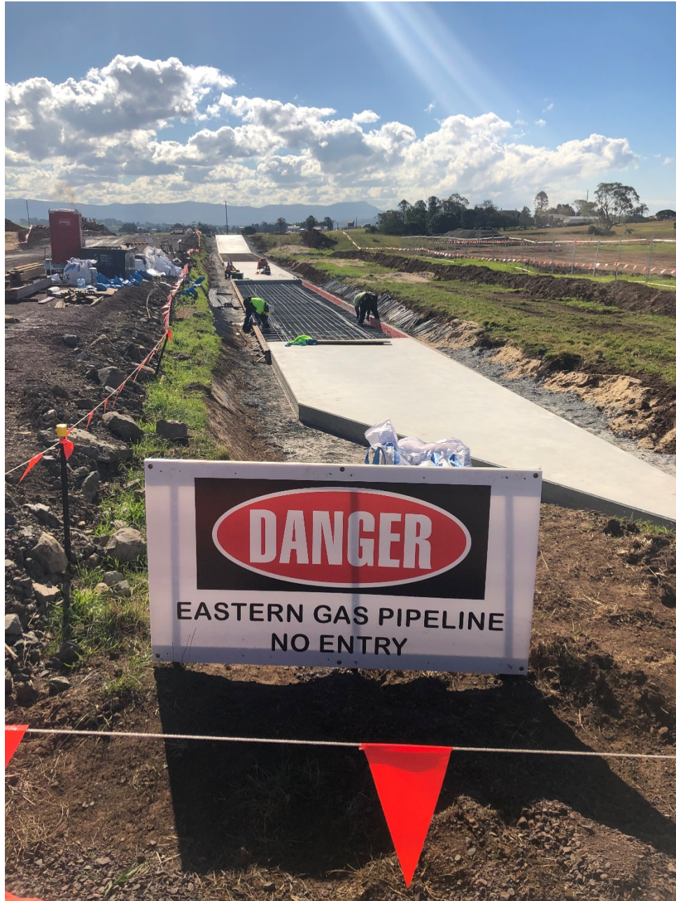
Figure 2-7: Eastern Gas Pipeline protection works
