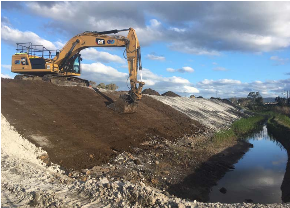
Figure 2-9: Progressive stabilisation of Fill 2 near Yallah
