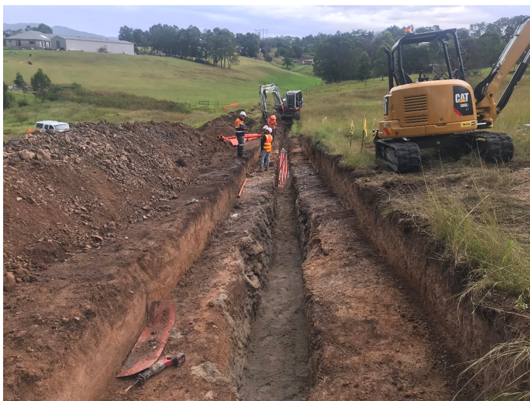
Figure 2-1: Installation of underground services in Cut 1
