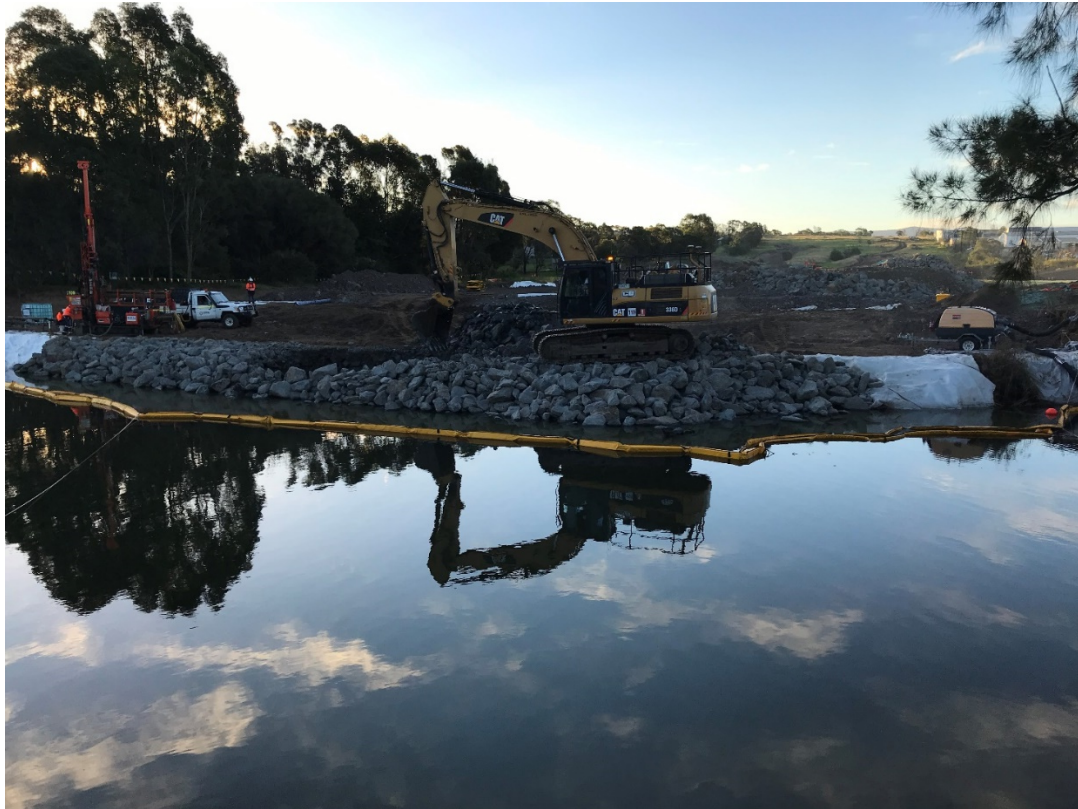
Figure 2-5: Construction of piling platform at Macquarie Rivulet
