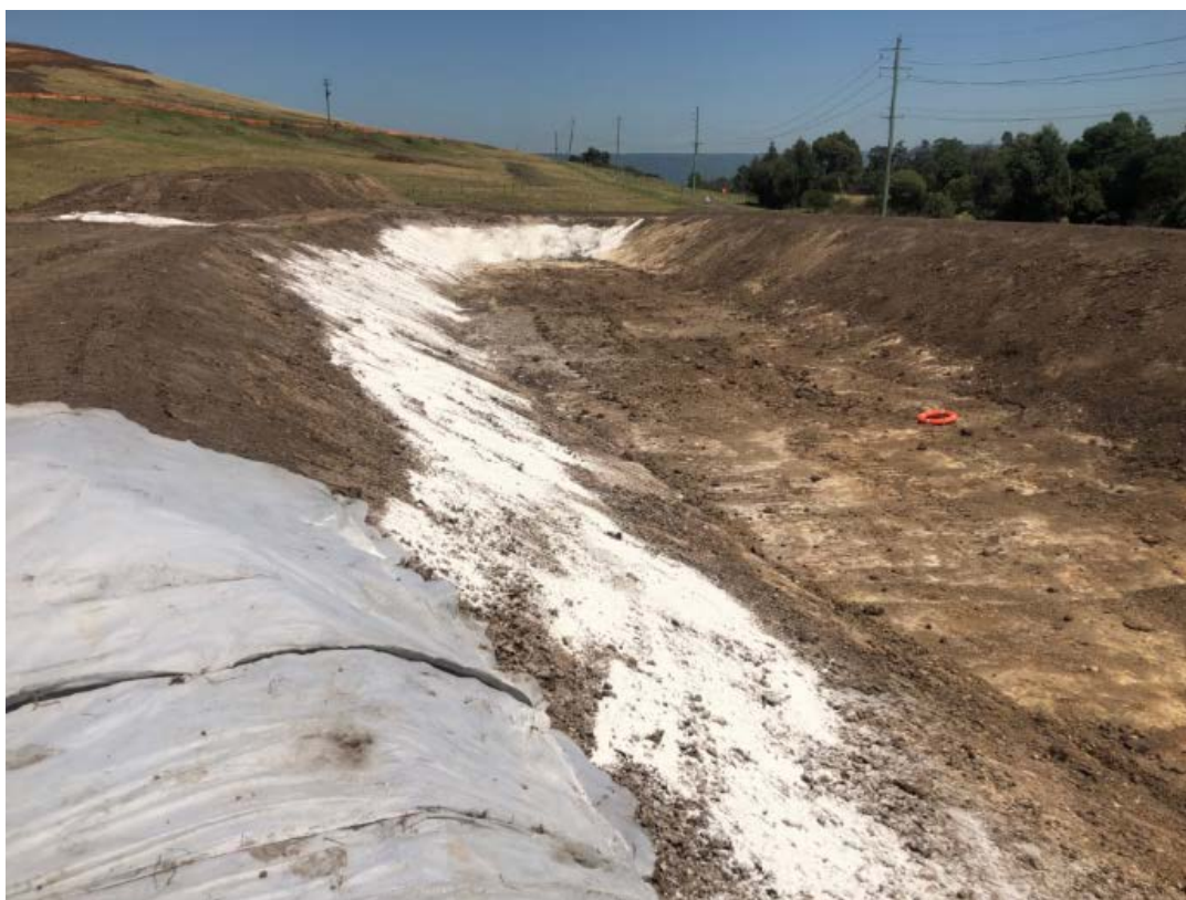
Figure 2-10: Installation of sediment basin in Cut 5 near Oak Flats Interchange, prior to earthworks commencing
