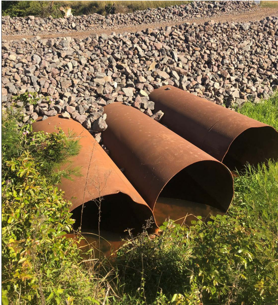
Figure 2-11: Temporary creek crossing at Frazers Creek #3
