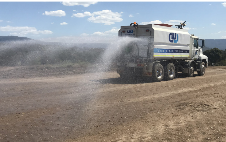
Water carts are used to suppress dust on active construction areas and unsealed roads.
