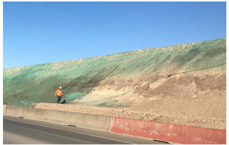
Hydromulching is used to quickly vegetate areas and suppress dust from exposed areas on the project.
