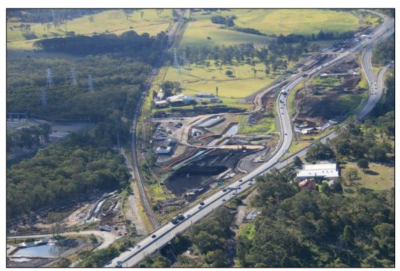
**Figure 3:** Aerial view of the northern portion of the project corridor in the vicinity of Yallah Road during late June 2019. Placement of imported fill materials, piling, utility adjustments and drainage works were in progress at this location.
