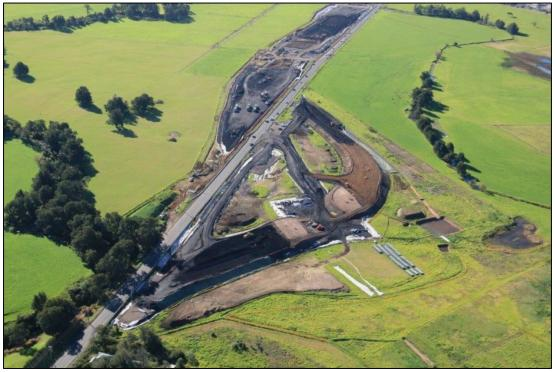
**Figure 2:** Aerial view of the central portion of the project corridor in the vicinity of the Illawara Highway during late June 2019. Placement of fill material was noted to be progressing well during the reporting period with a high standard of environmental management evident.
