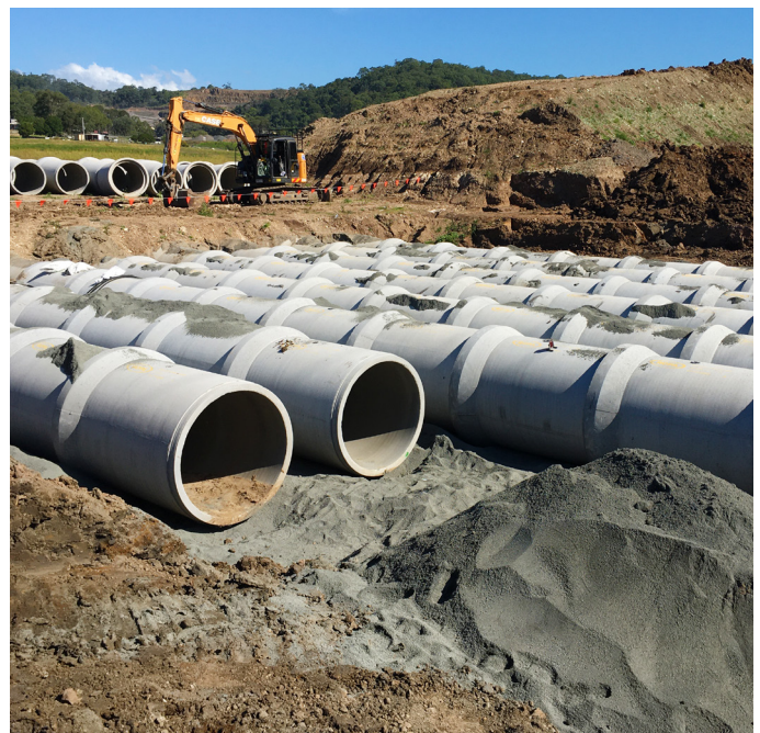
Drainage work under the East West Link - April 2020
