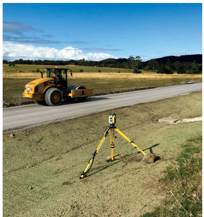
Placing pavement on the southbound entry ramp at Tongarra Road - June 2020
