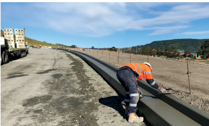
Building kerb on the new Croome Road – June 2020
