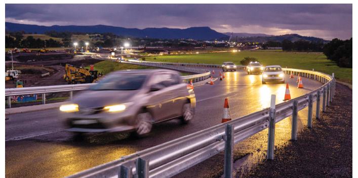
First cars to drive over the new bridge into Albion Park
