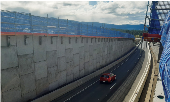
Princes Motorway at Yallah – May 2020
