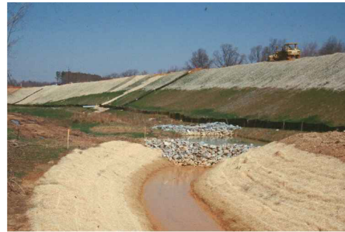
PHOTO 2 - PROGRESSIVE STABILISATION OF BATTERS AS WORKS PROGRESS
