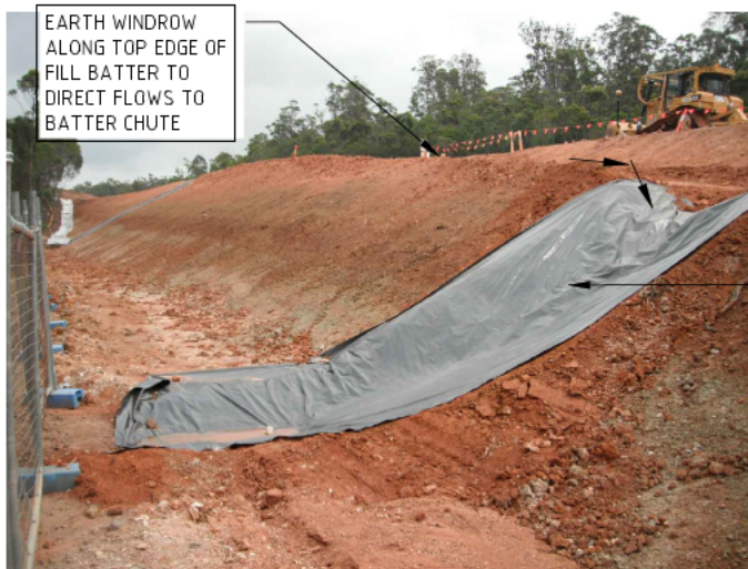
PHOTO 4 - EXAMPLE OF BATTER CHUTE
