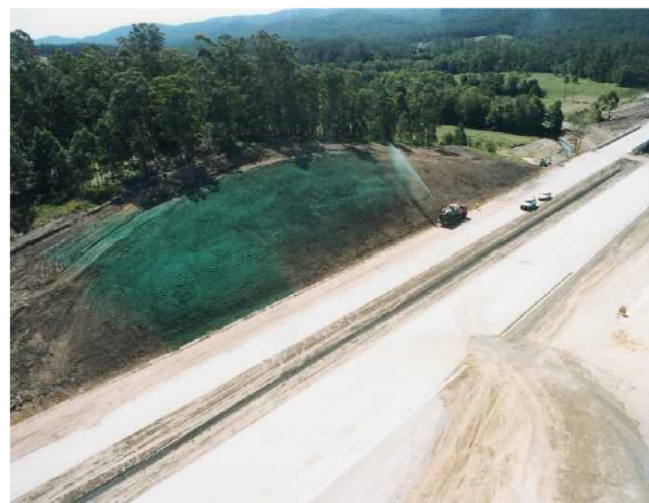
PHOTO 5 - TEMPORARY STABILISATION OF BATTERS WITH POLYMER
