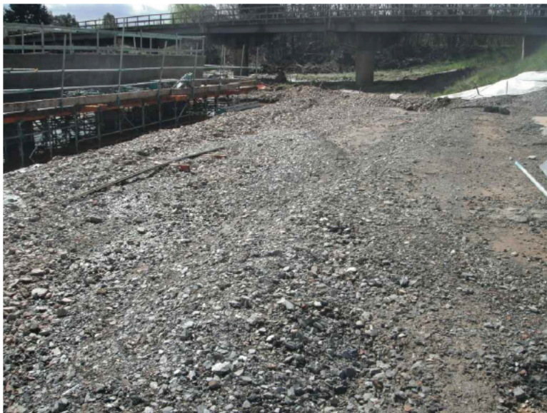
PHOTO 6 - EXAMPLE OF A PILING PLATFORM STABILISED SURFACE
