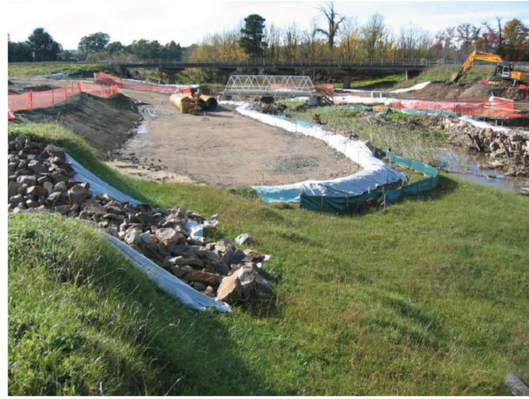
PHOTO 7 - EXAMPLE OF A PILING PLATFORM WITH ROCK FILTER BUND
