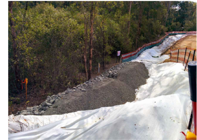
PHOTO 3 - EXAMPLE OF ROCK FILTER DAM AND SUMP
