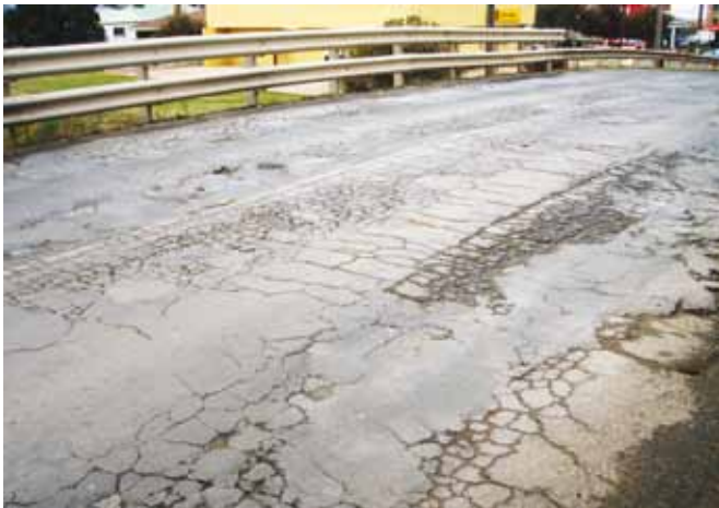
Rough pavements reduce traveller comfort and result in increased vehicle running costs.
