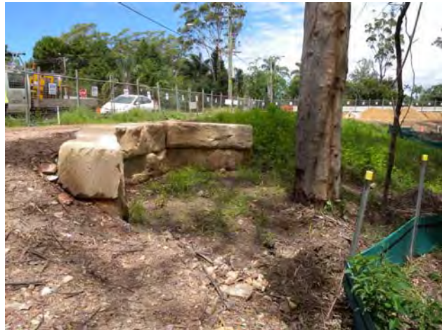
Figure 12 Example of informal low retaining wall
