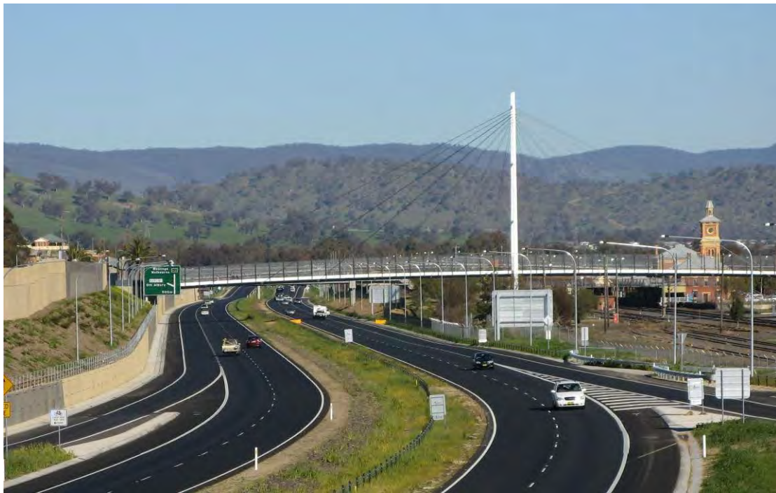
Figure 4-7 The difference between avoiding and mitigating impacts Locating the road alignment at the bottom of the hill and in redundant land alongside the rail line helped avoid landscape character and visual impacts. The residual noise impacts and the impacts of crossing the road still had to be mitigated but the mitigation measures of walls and bridges were well designed and integrated architecturally with the whole project.
