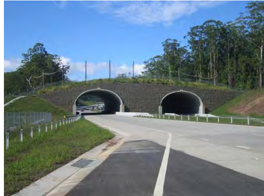
This fauna overpass - through its planting, proportions and use of local stone around the arches - has been designed to integrate with the forest setting and provide a visually acceptable element on the road corridor.
