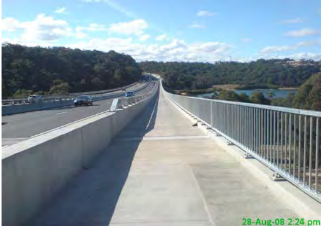
Figure 5 Alfords Point Bridge
