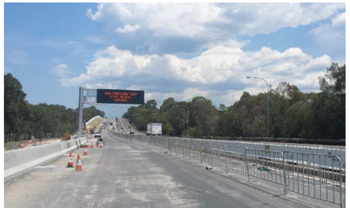
Installation of the new electronic message sign
