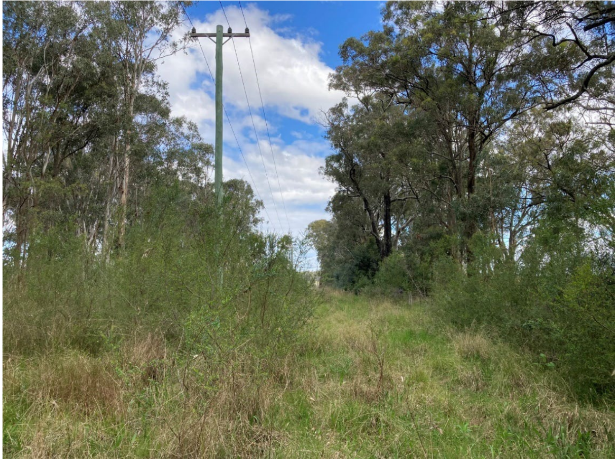
Figure 2.4 Electrical transmission line and vehicle track facing south.
