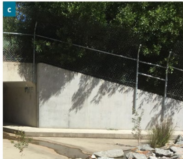
Figure 9 Example of koala/fauna grid with fenced return (left) and wing wall drop-down 21 (right)
