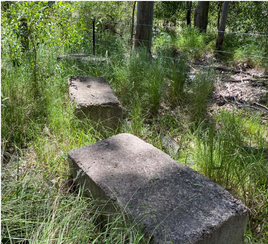
Figure 42 Concrete blocks placed along fence line to prevent access to property from Appin Road.
