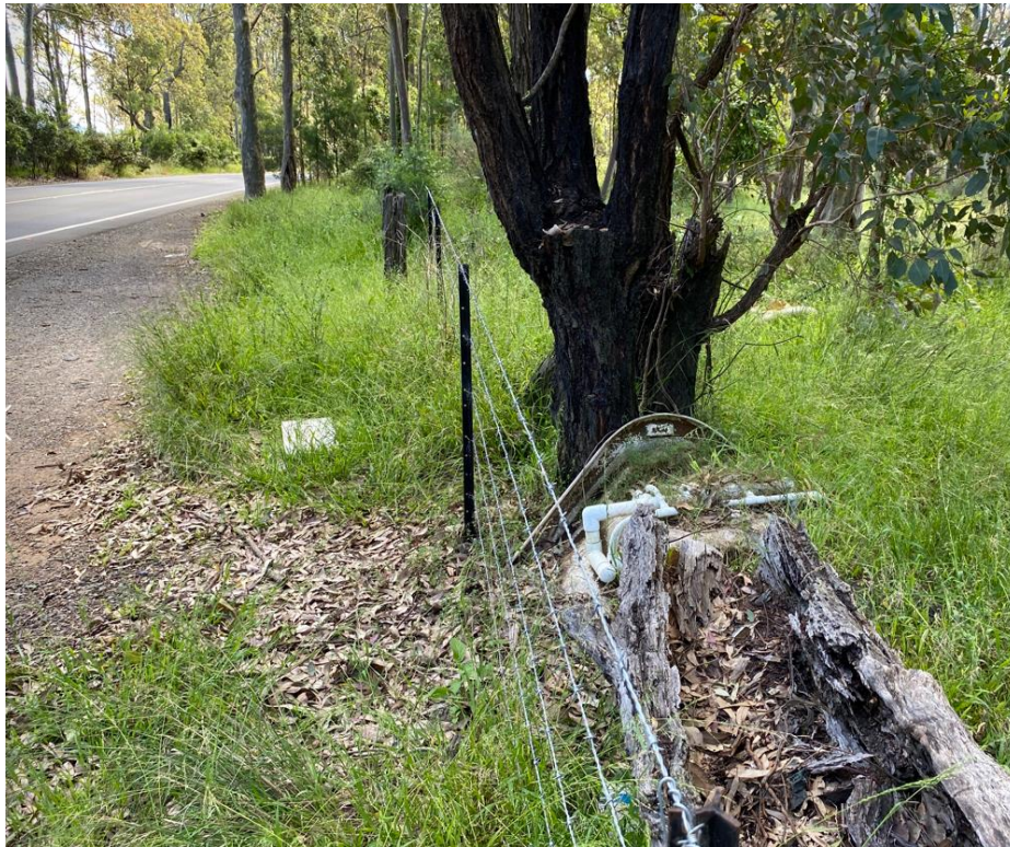
Figure 31 New fencing immediately adjacent to older fencing. Rubbish dumped along fence line. Hardstand area from previous road works and evidence of pavement materials stockpiled adjacent to fence line.
