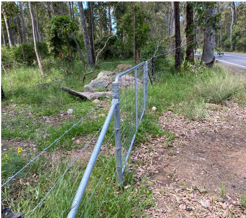
Figure 30 Access gate for electrical maintenance, bushfire track access and access to property along fence line. Evidence of dumped rubbish scattered along fence line.
