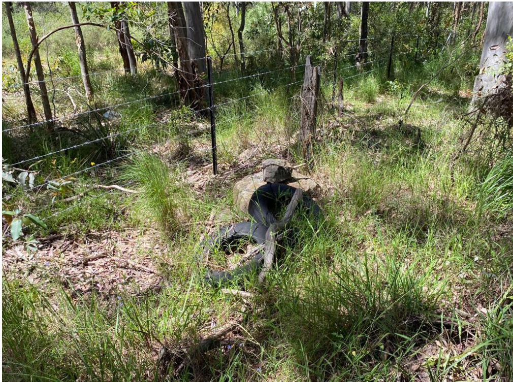
Figure 43 New fencing installed adjacent to disused fencing. Rubbish dumped along fence line. Communications services along fence line.
