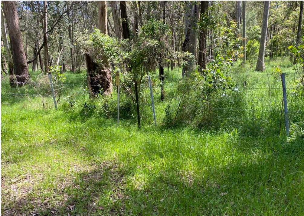
Figure 50 Communications marker posts indicating services adjacent to fence line.
