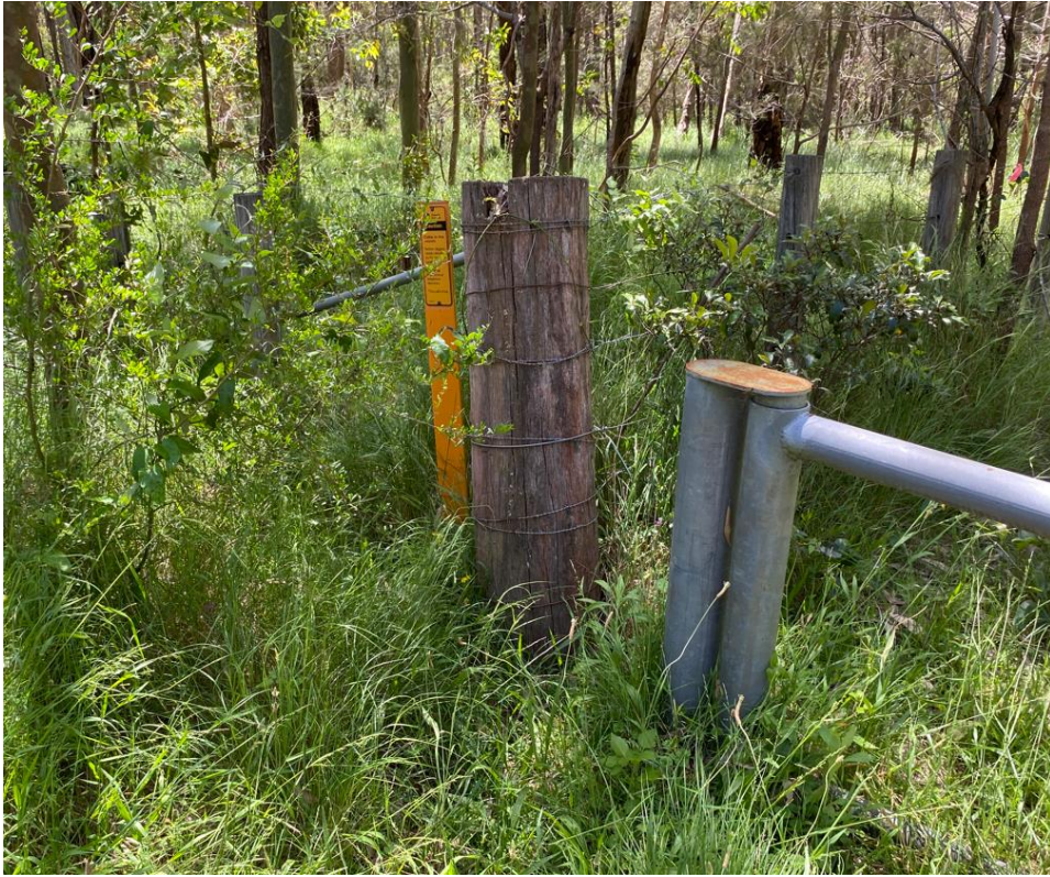
Figure 53 Communications marker post indicating communications services adjacent to fence line.
