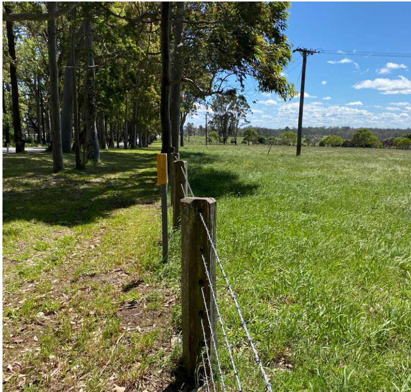
Figure 23 Cleared access to fence line for maintenance. Communications markers indicating underground communications line. Overhead wires adjacent to fence line. Grazing pastureland within fencing.
