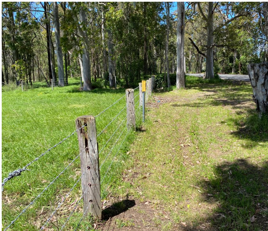
Figure 22 Communications marker posts indicating presence of communications services along fence line.
