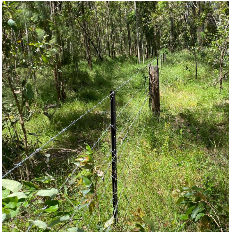
Figure 27 New fencing installed immediately adjacent to existing timber fencing.
