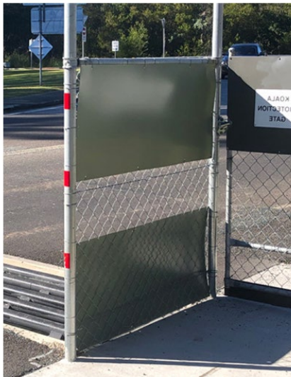
Figure 9 Example of koala/fauna grid with fenced return (left) and wing wall drop-down 21 (right)
