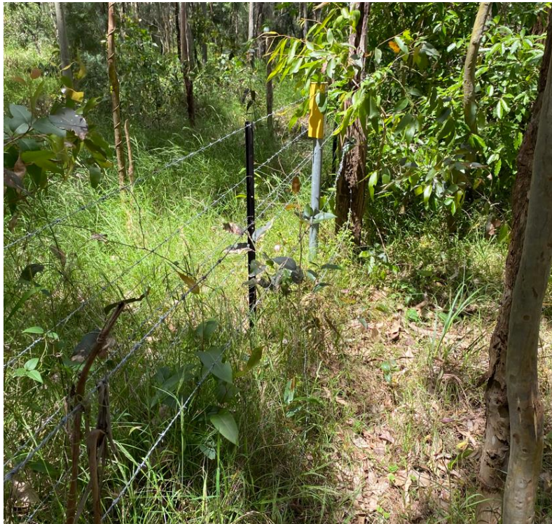
Figure 47 New fence installed adjacent to disused fencing. Communications marker post indicating communications services along fence line.
