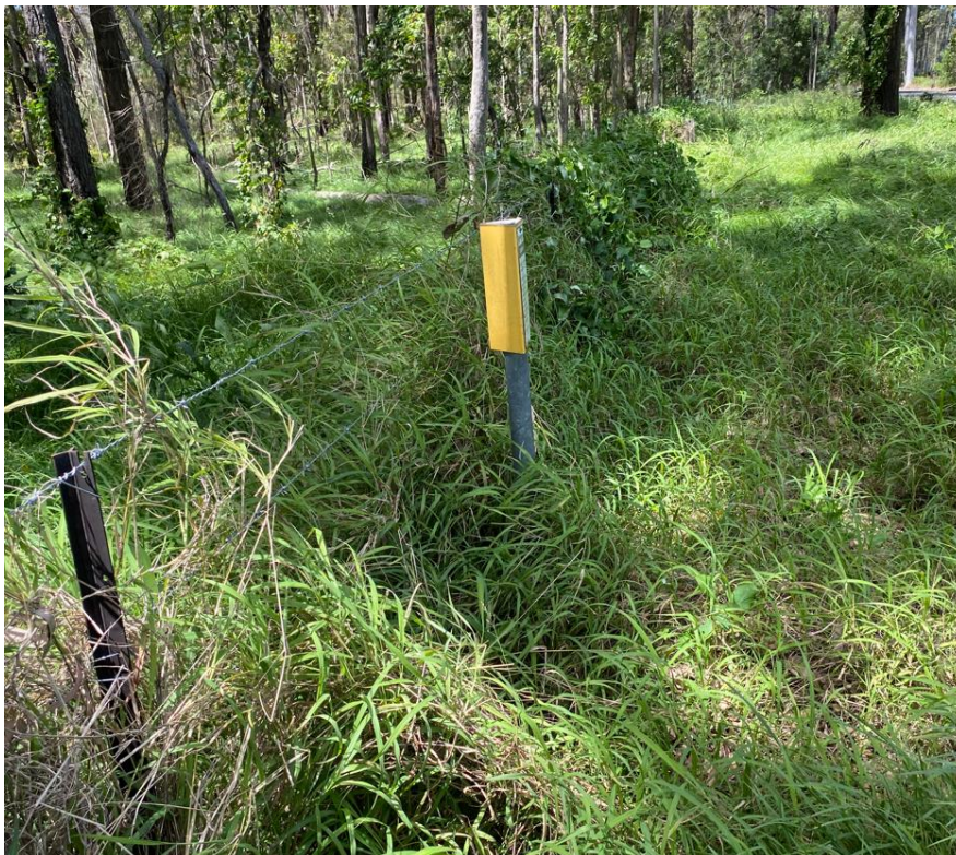
Figure 26 Communications marker indicating presence of services along route of fence line.
