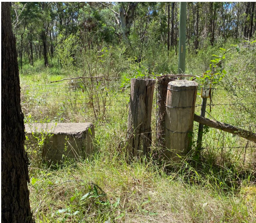
Figure 5 Existing fence line and strainer post with wires removed. Concrete blocks placed to prevent access from Appin Road.
