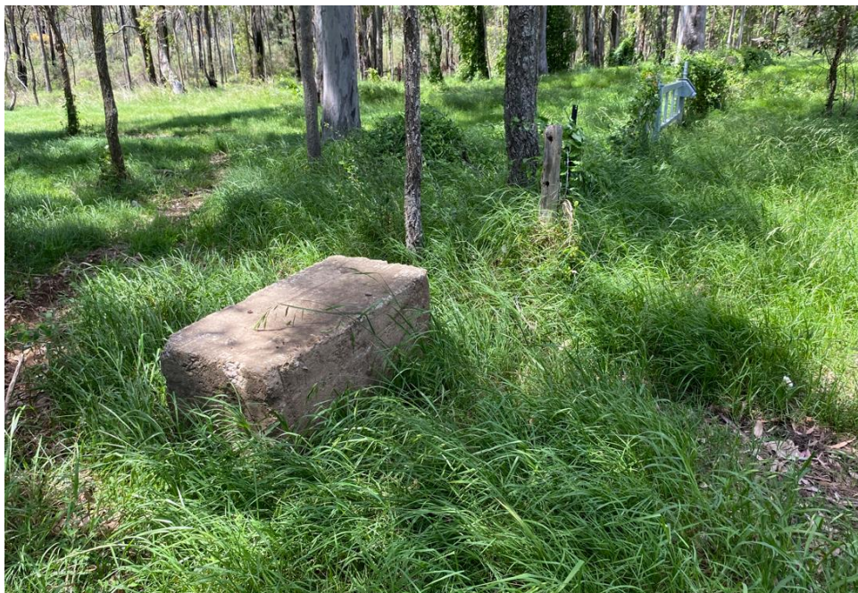
Figure 24 Overgrown fence line. Wires cut and concrete blocks placed to prevent access from Appin Road. Access gate installed along fencing route for electrical maintenance and bush fire access.
