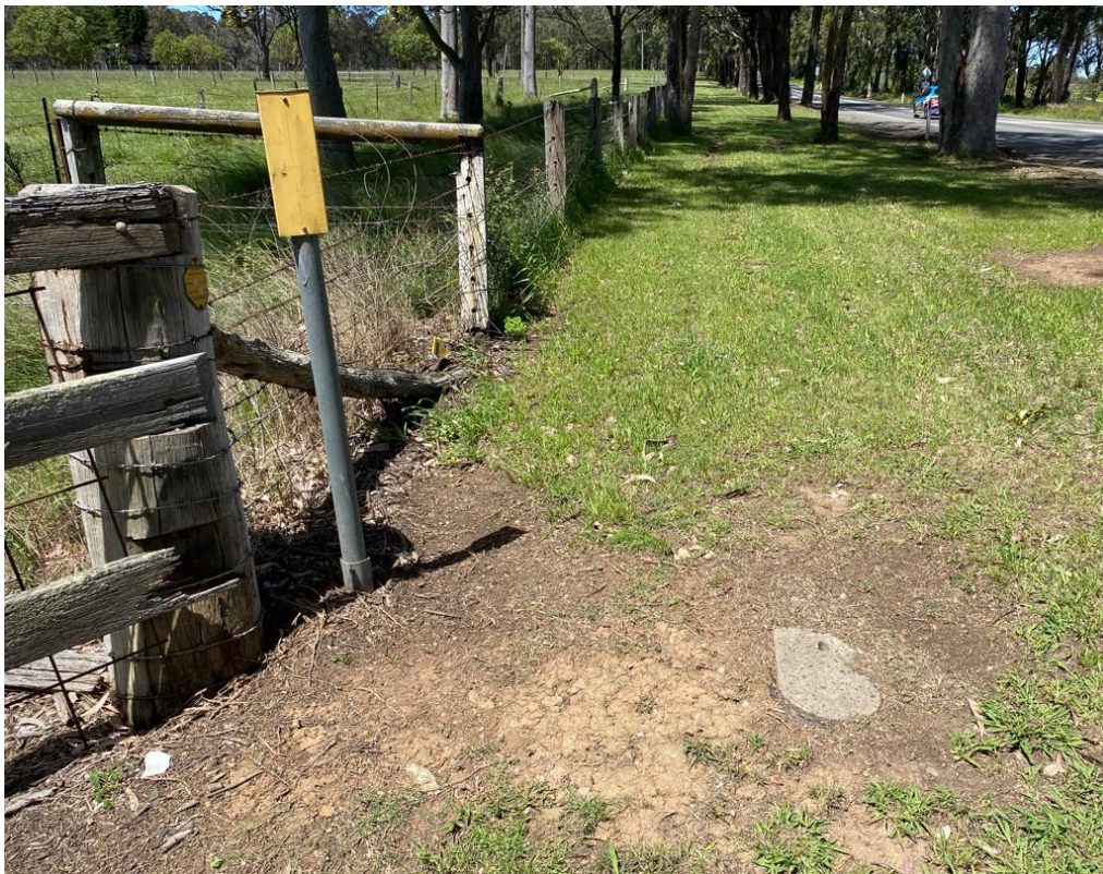
Figure 17 Communications trenching and access pit along fence route.
