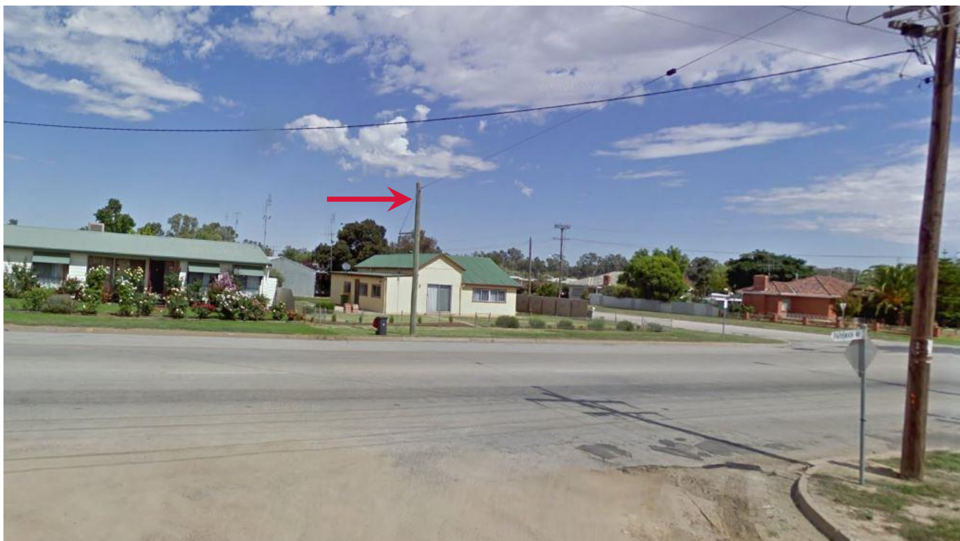
Figure 3-3 Electricity stay pole to be removed and replaced (looking south-west from Parkman Ave)
