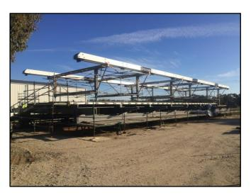
Truss span two being assembled in the Koondrook site compound.
