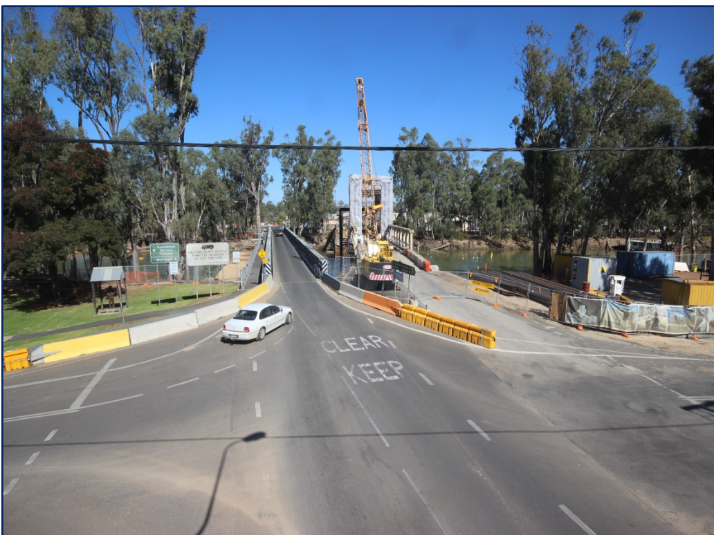
Work site on the NSW side of the bridge.
