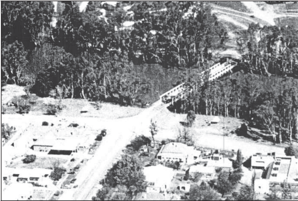
Figure 10: Bridge over the Murray River at Barham (source: Barham-Koondrook Historical Society 2004)
