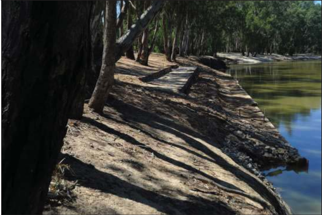
Plate 7: Retaining walls east of the Barham Bridge, facing 125° (Photo: B. Grinter 12/12/2014)
