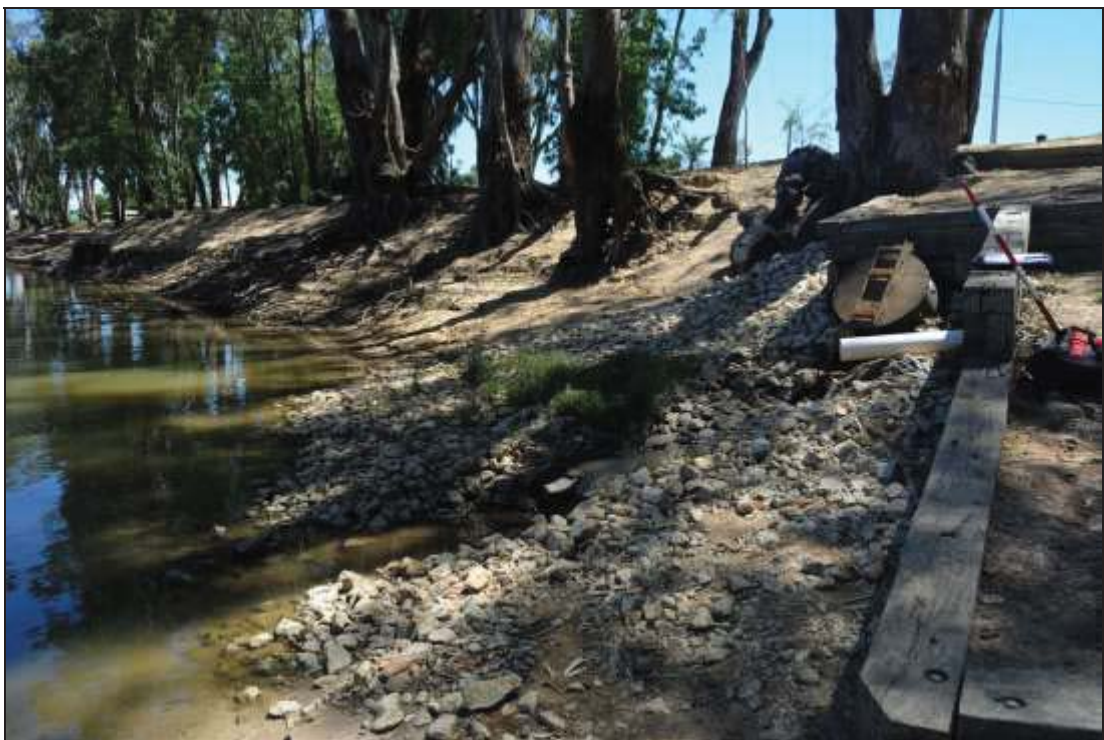
Plate 8: Drain disturbance, facing 340° (Photo: B. Grinter 12/12/2014)
