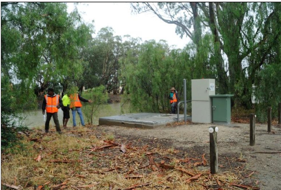
Plate 4: Pumping station, facing 90° (Photo: J.Bell 13/1/15)
