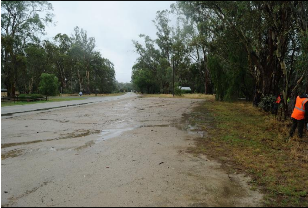
Plate 1: Road side verge at Murray Parade, facing 310° (Photo: J.Bell 13/1/15)
