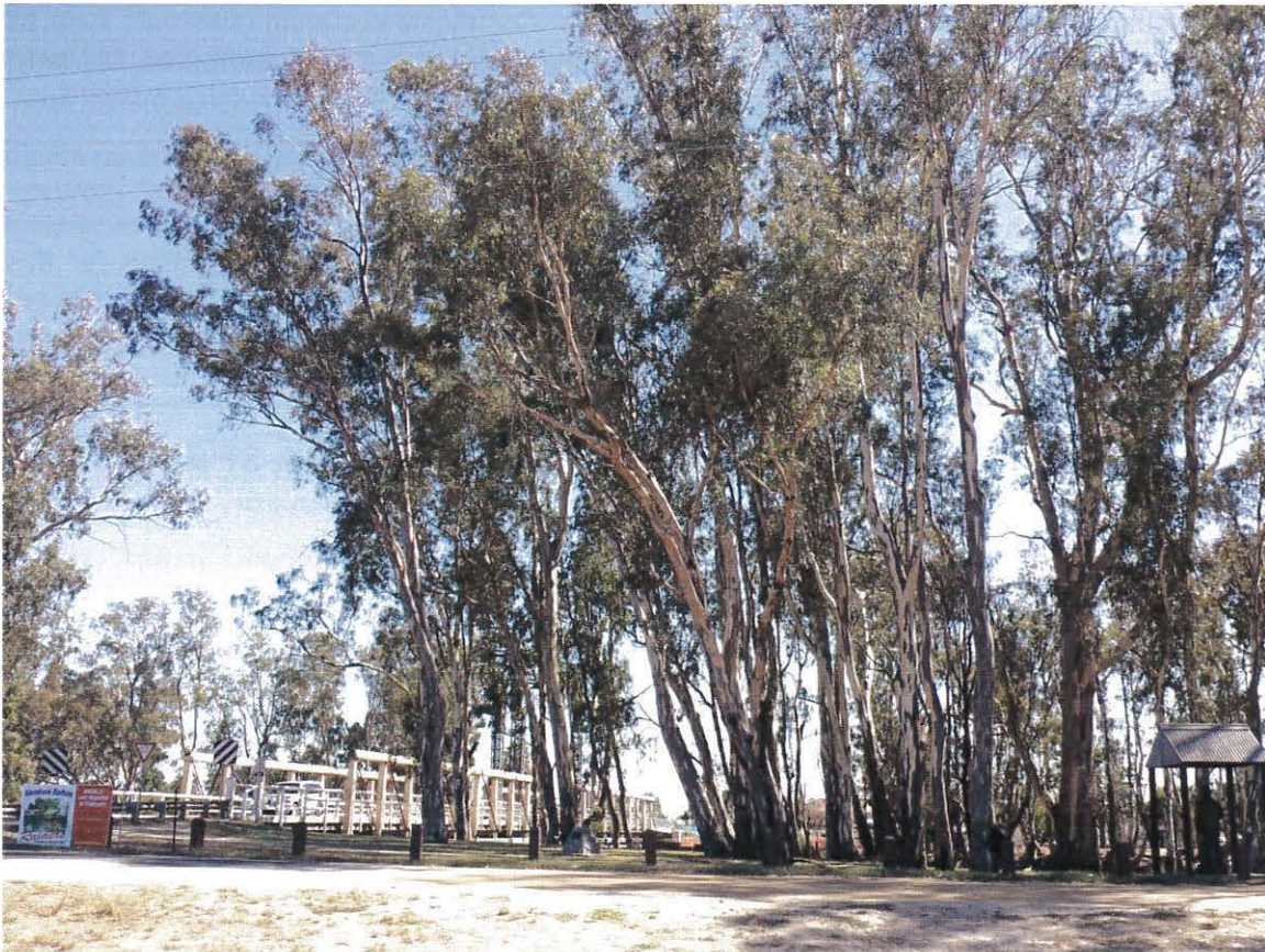
Figure 4-2 Looking north towards the Barham Bridge along the proposed temporary crossing location
