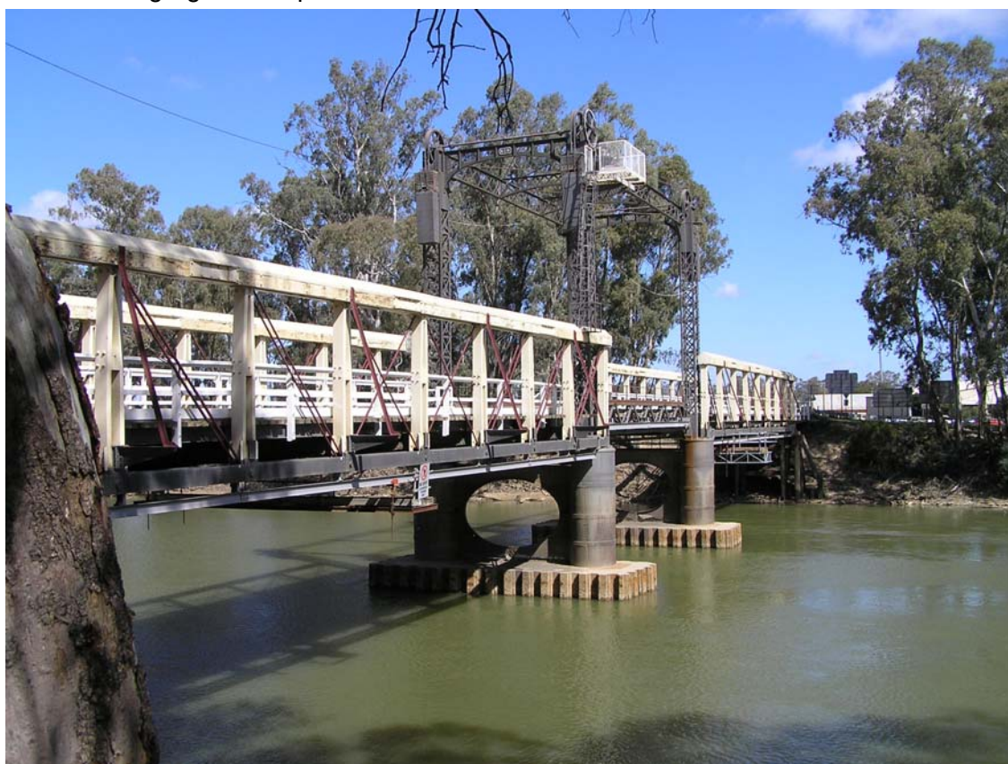
Figure 11: General View of Barham Bridge looking south (RMS).
