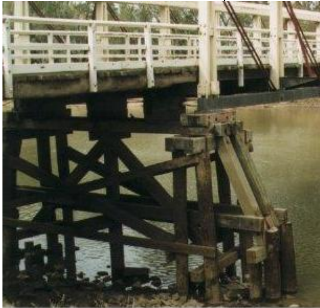
Figure 17: View of the timber trestle Pier 4.
