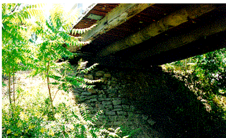
Figure 28: Abutment A at St Albans Bridge.
