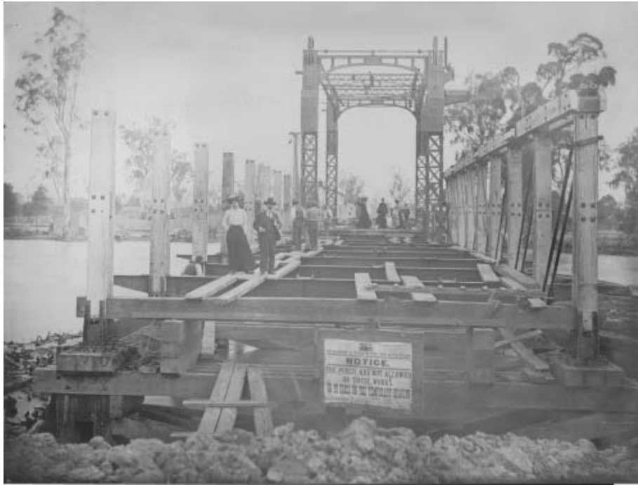
Figure 6: View of the Bridge during construction in mid 1904 with lift span in place. The near side span has the right hand truss complete, but left hand truss is still under construction. The deck cross-members of the near side span are in place, but not decking (University of Melbourne Archives, UMA/I/6290).
