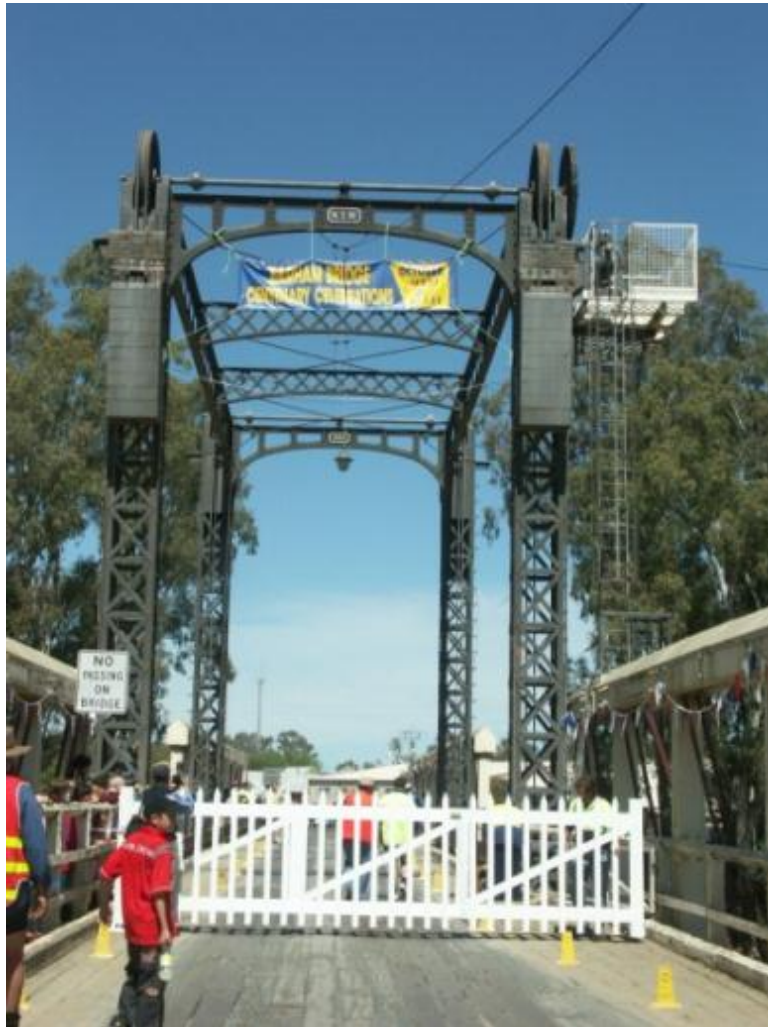
Figure 8: Decorative gate set up on bridge for Centenary celebrations, October 9 th and 10 th , 2004, note access ladder right side of lift span first attached to bridge in 1923 and replaced at regular intervals.
