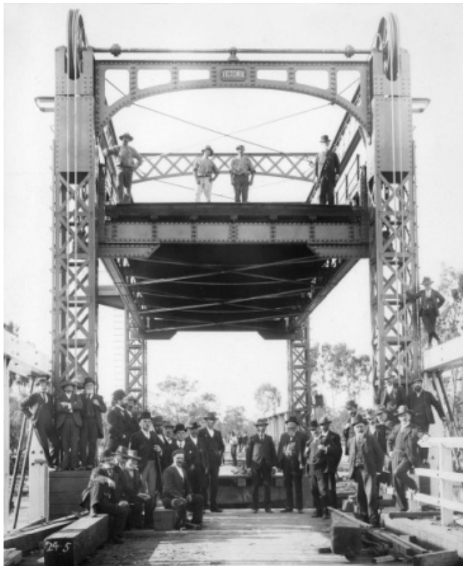
Figure 7: Lift span raised during the official opening of Barham Bridge in September 1904 (University of Melbourne Archives, BWP/23843).
