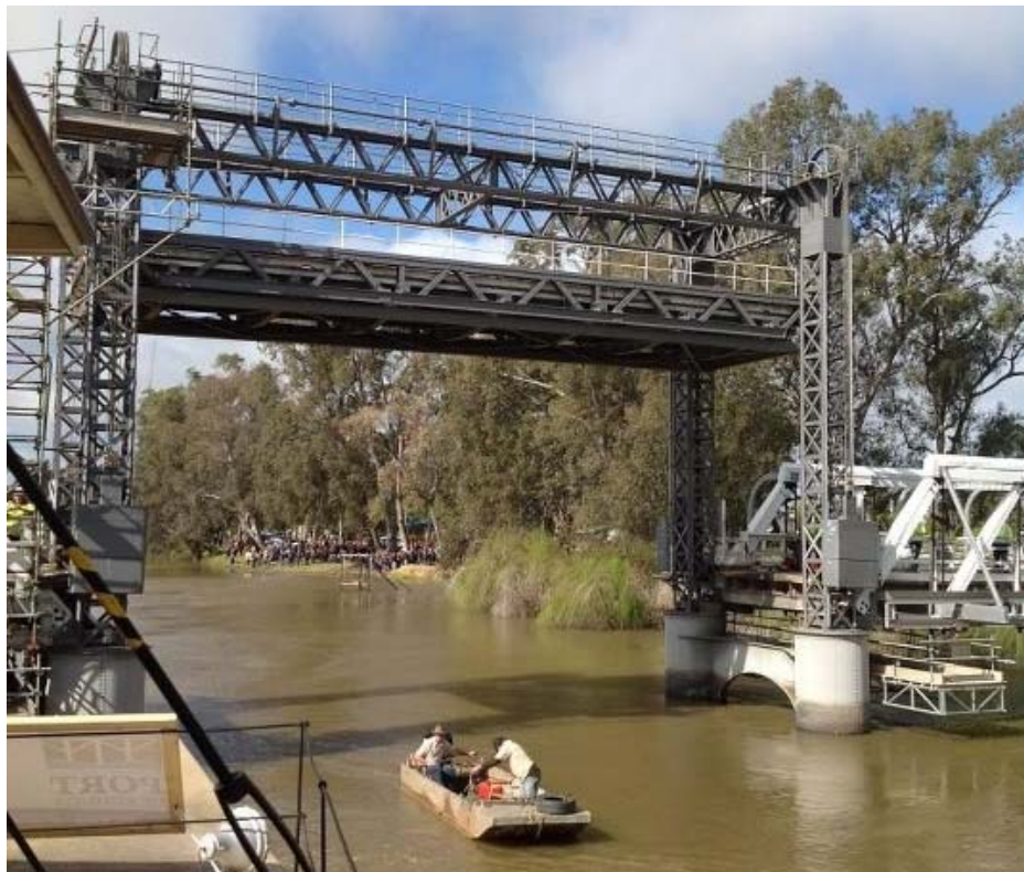
Figure 10: A test left undertaken in 2012 after repair works (RMS Bridge File).
