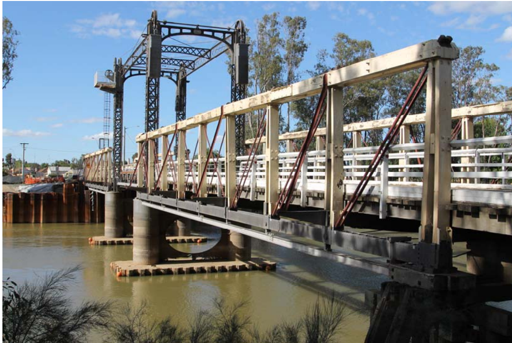
Figure 20: View of southern truss span (Span 4).
