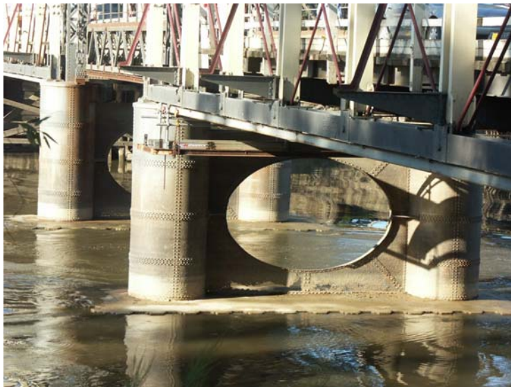
Figure 18: View of the iron Piers 2 and 3.
