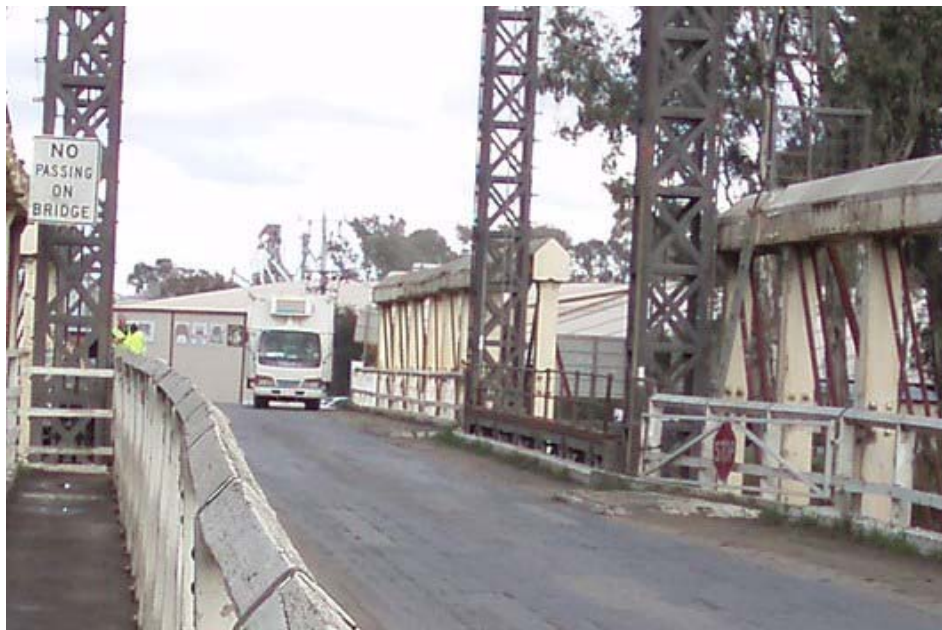
Figure 21: View of deck on lift and truss spans.
