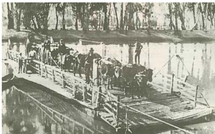
Figure 4: Punt unloading cattle at Barham-Koondrook (Source: Grant 1970).
