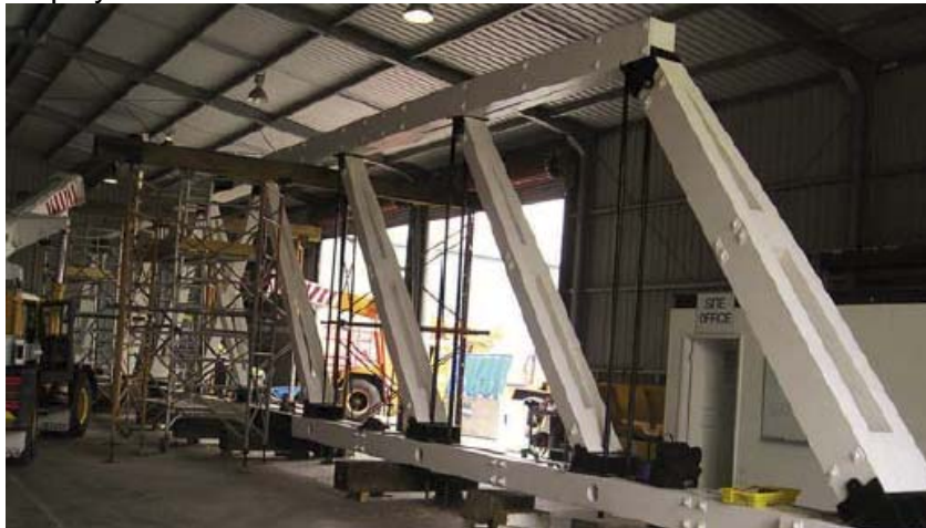
Figure 32: Replacement truss span of Hinton Bridge under construction in 2006.
