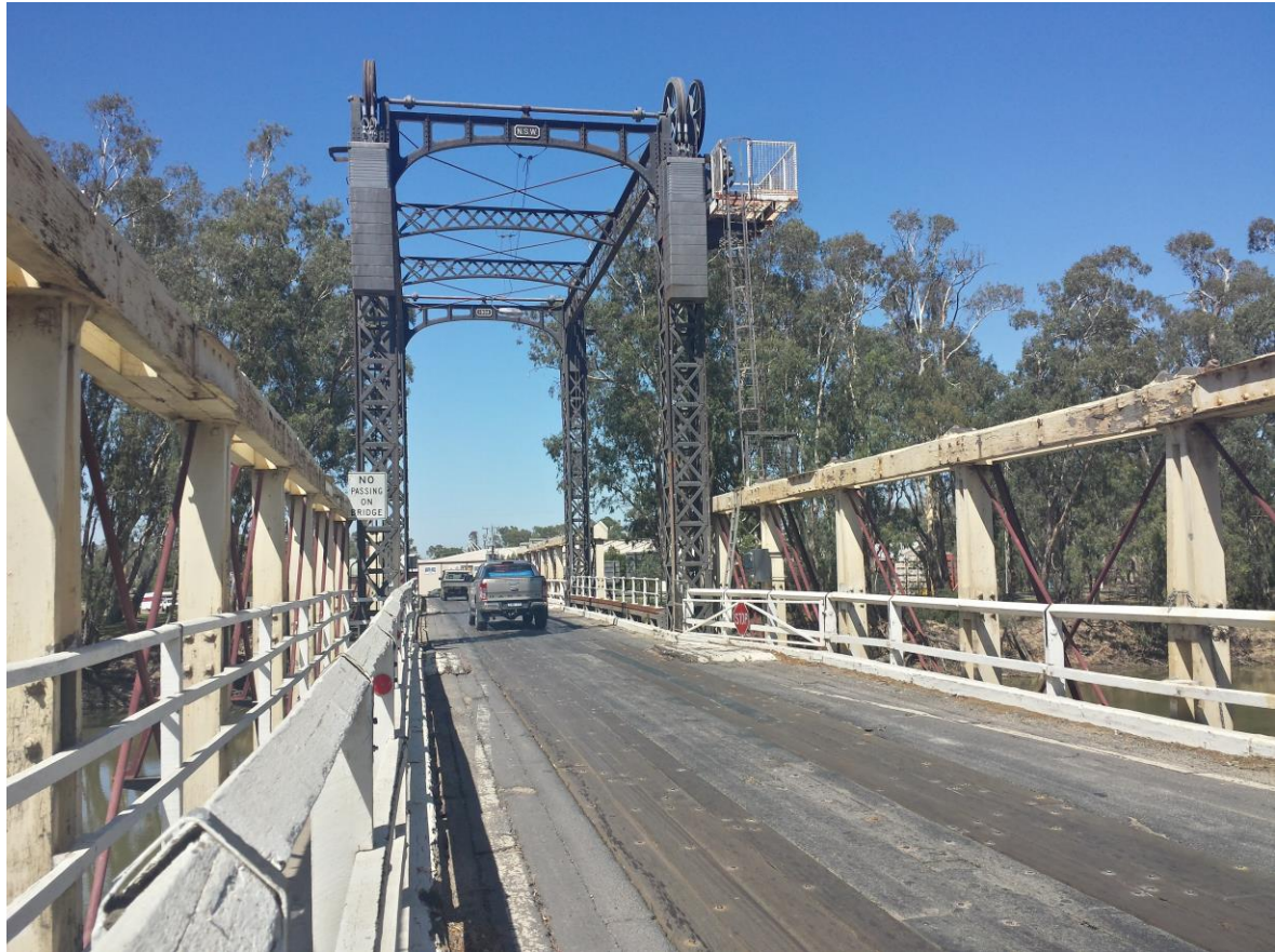
Figure 2-2 Photo of the lift span of the Barham-Koondrook Bridge
