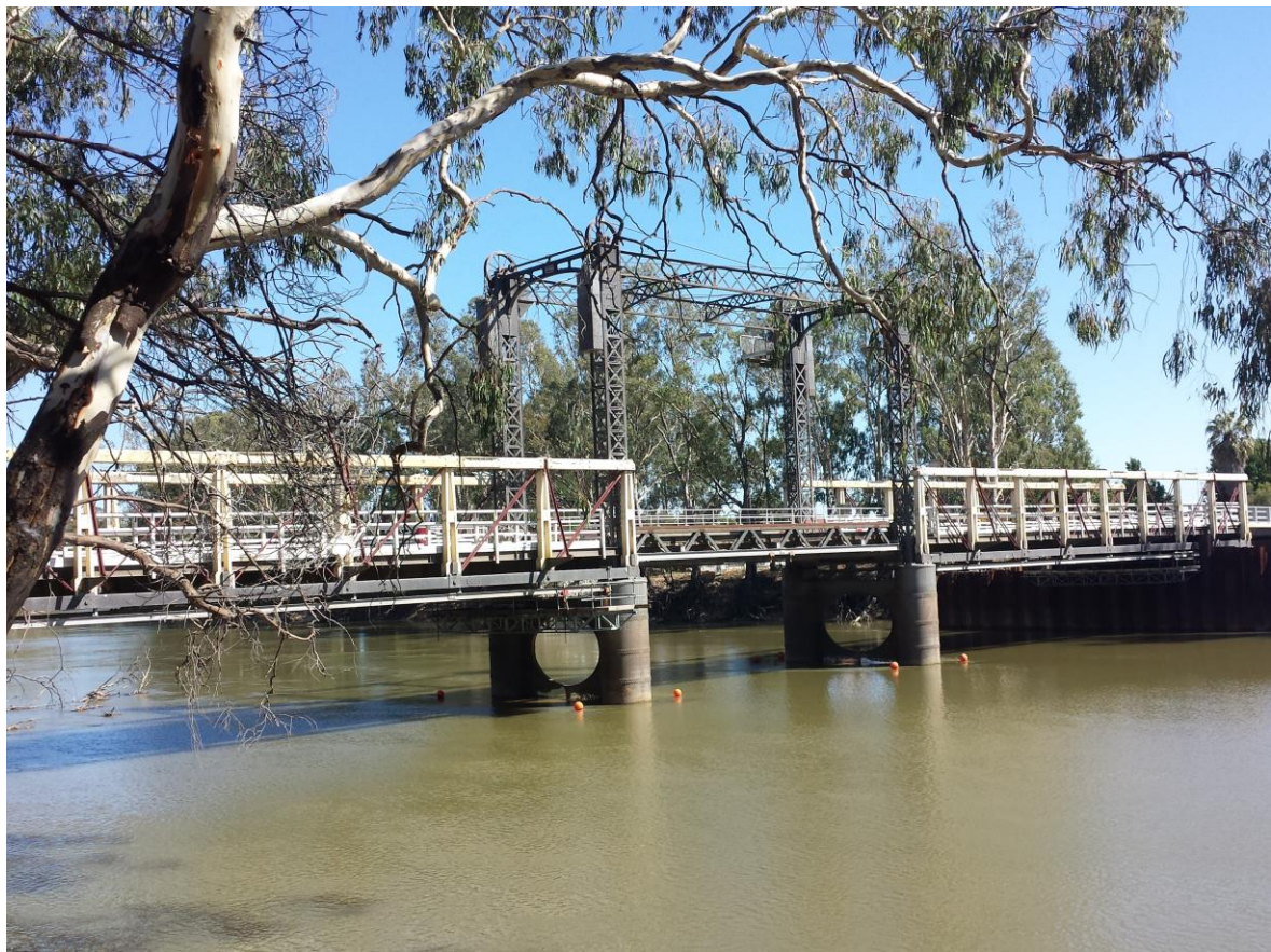
Figure 2-1 Photo of the Barham-Koondrook Bridge
