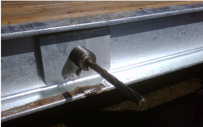
Figure 34: Detail of the tension rod
