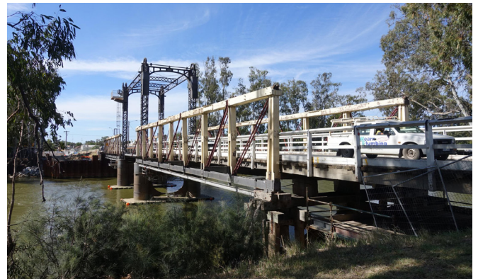
Figure 26: The De Burgh truss was built in a short period of time between 1899 and 1905
