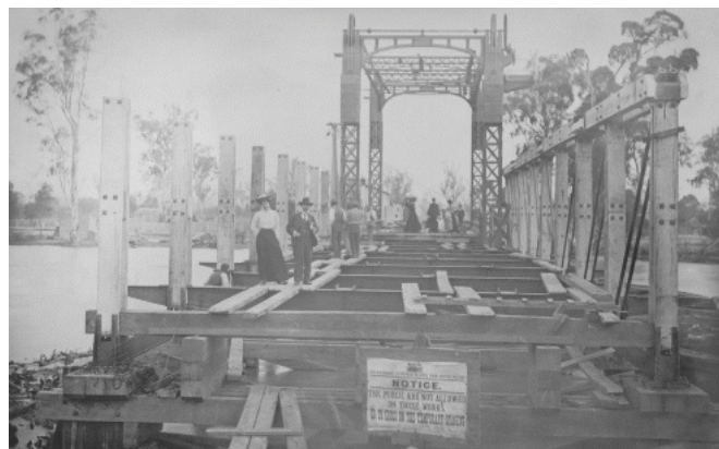
Figure 11: Barham Bridge Construction (Source: Kerang New Times, 1904, The Barham-Koondrook Historical Society)
