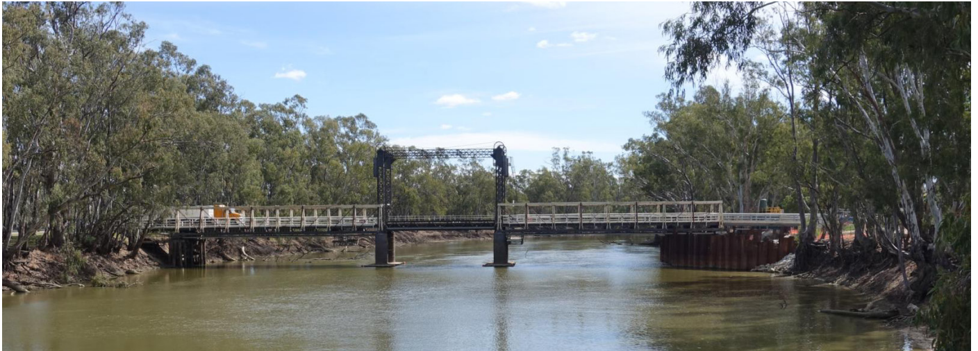
Figure 4: View of the bridge from the Barham side of the river. The shoreline vegetation strongly frames the bridge structure
