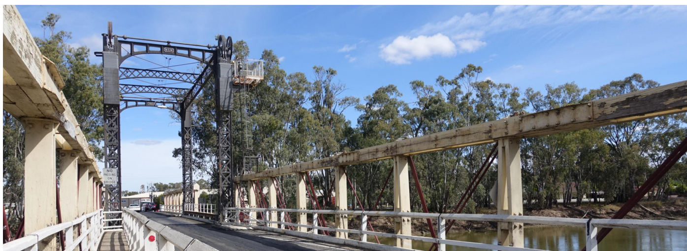
Figure 6: View looking towards the tower of the lifting span that forms an important element of the bridge
