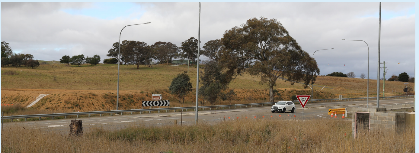
View of the Kaveney's Road intersection from the north west towards the Barton Highway. Stage 1 of duplication will stop before Kaveney's Road intersection.
