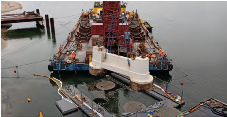
Headstocks being removed from the Clyde River as part of bridge removal work.
