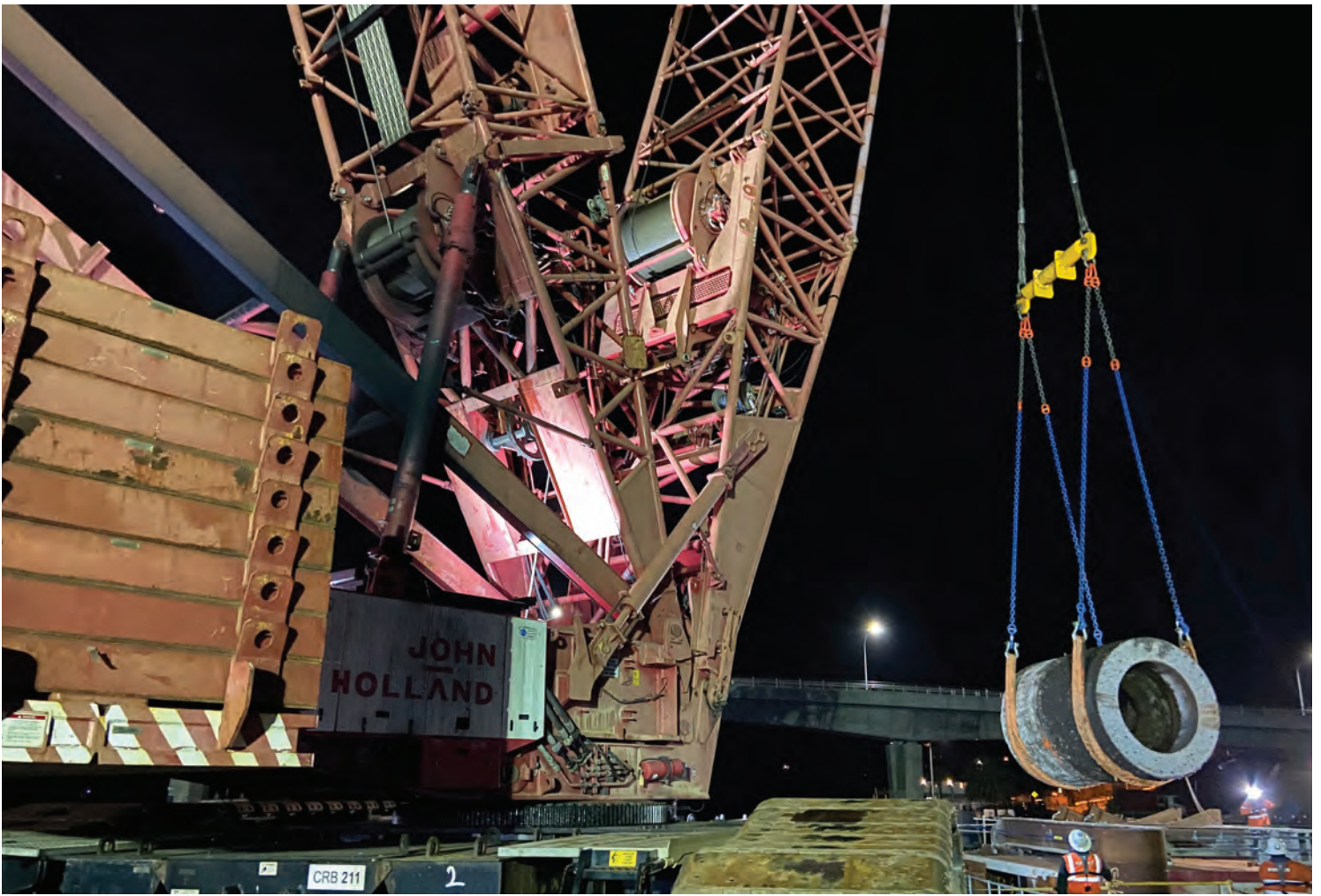
The concrete piles of the existing bridge are cut into pieces weighing between 50-113 tonnes and are removed using a crane.
