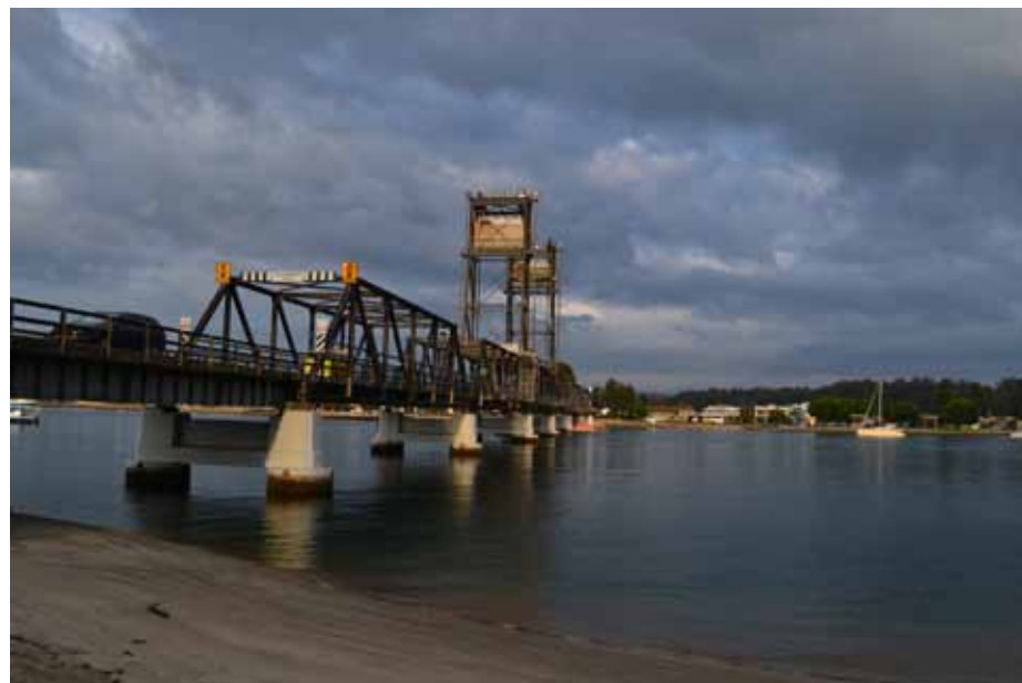
Figure 2.1 The liftspan towers are a dominant feature of the existing bridge. Source: Aurecon.
