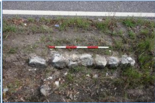
Plate 6.9 Stone gutter at Scenic Hill (CRSH 4)
