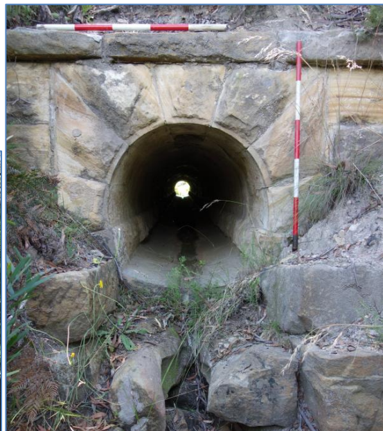
Plate 6.11 Sandstone culvert (CRC 23) which runs under Chifley Road at southern end of Clarence road over rail bridge section
