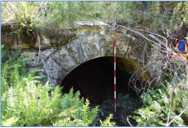
Plate 6.8 Sandstone culvert at Dargans Creek (CRC 2)
