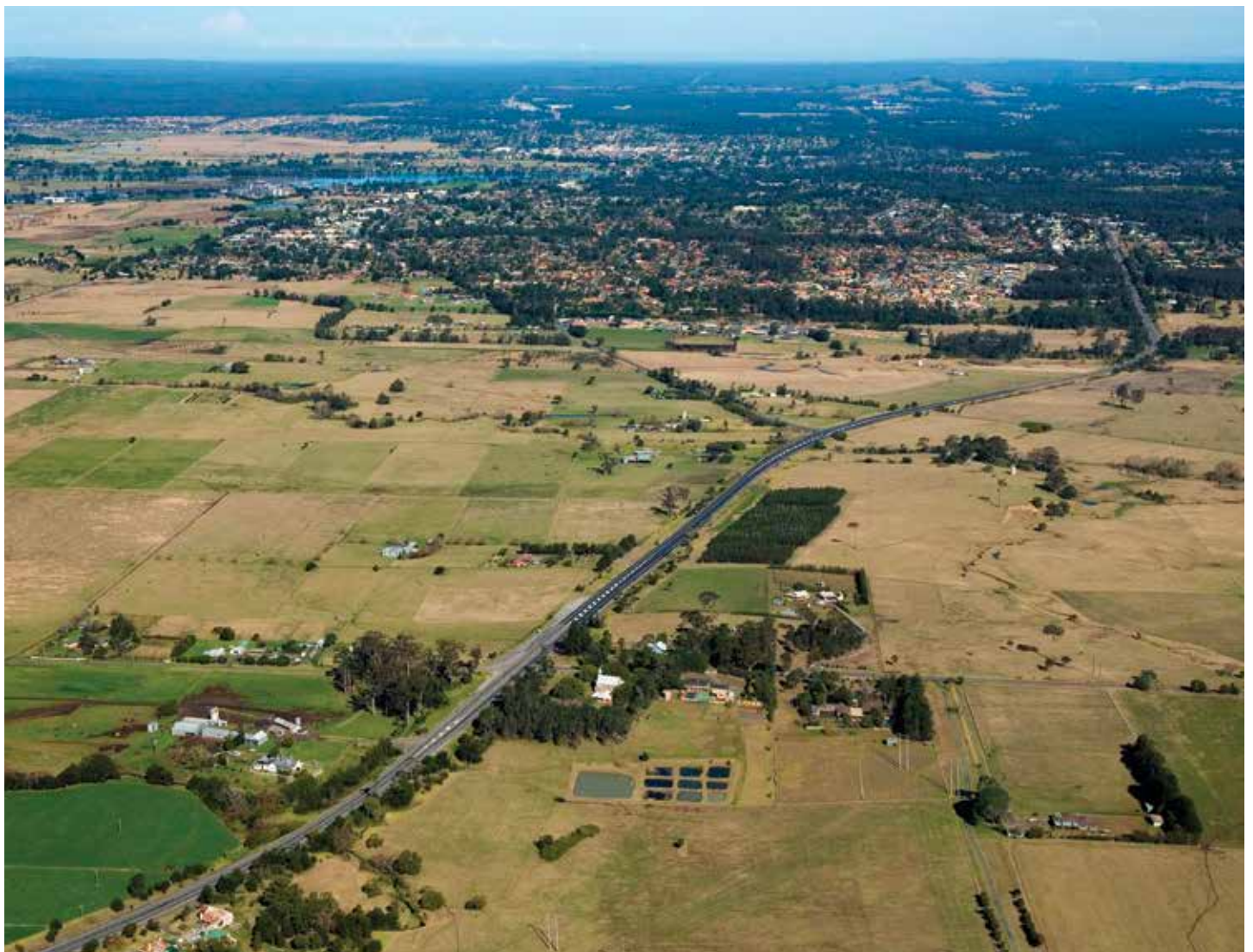
View of the Princes Highway at Meroo Meadow, looking towards Bomaderry
