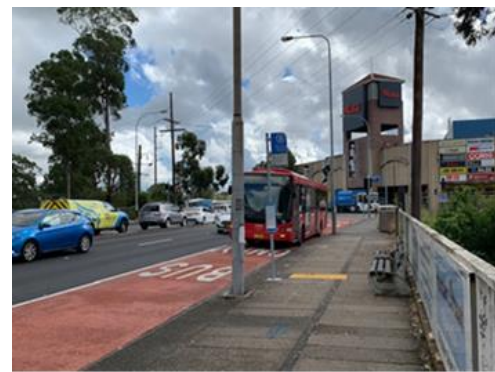
After the upgrade - bus only lane extended
