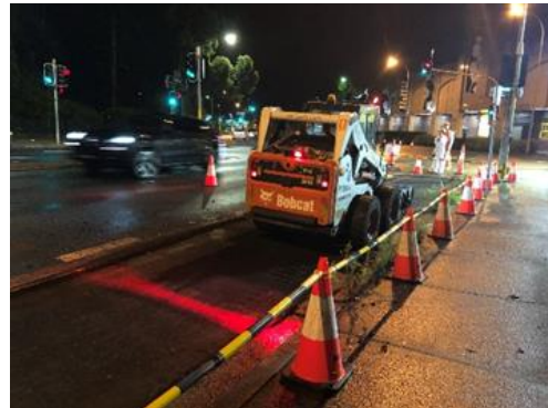
During night work - road asphalting
