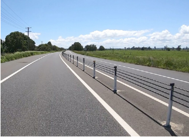
Example of the median safety barrier proposed at various locations on Big River Way
