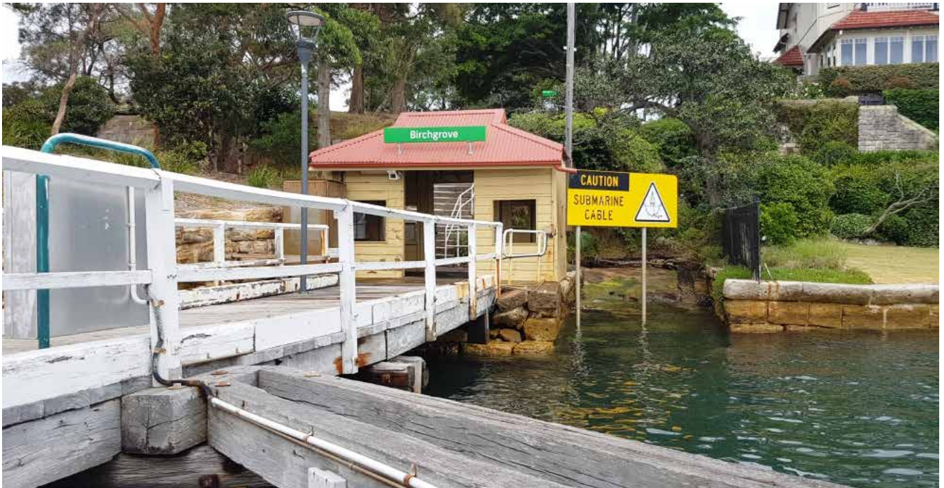
The existing wharf and waiting shed at Birchgrove Wharf
