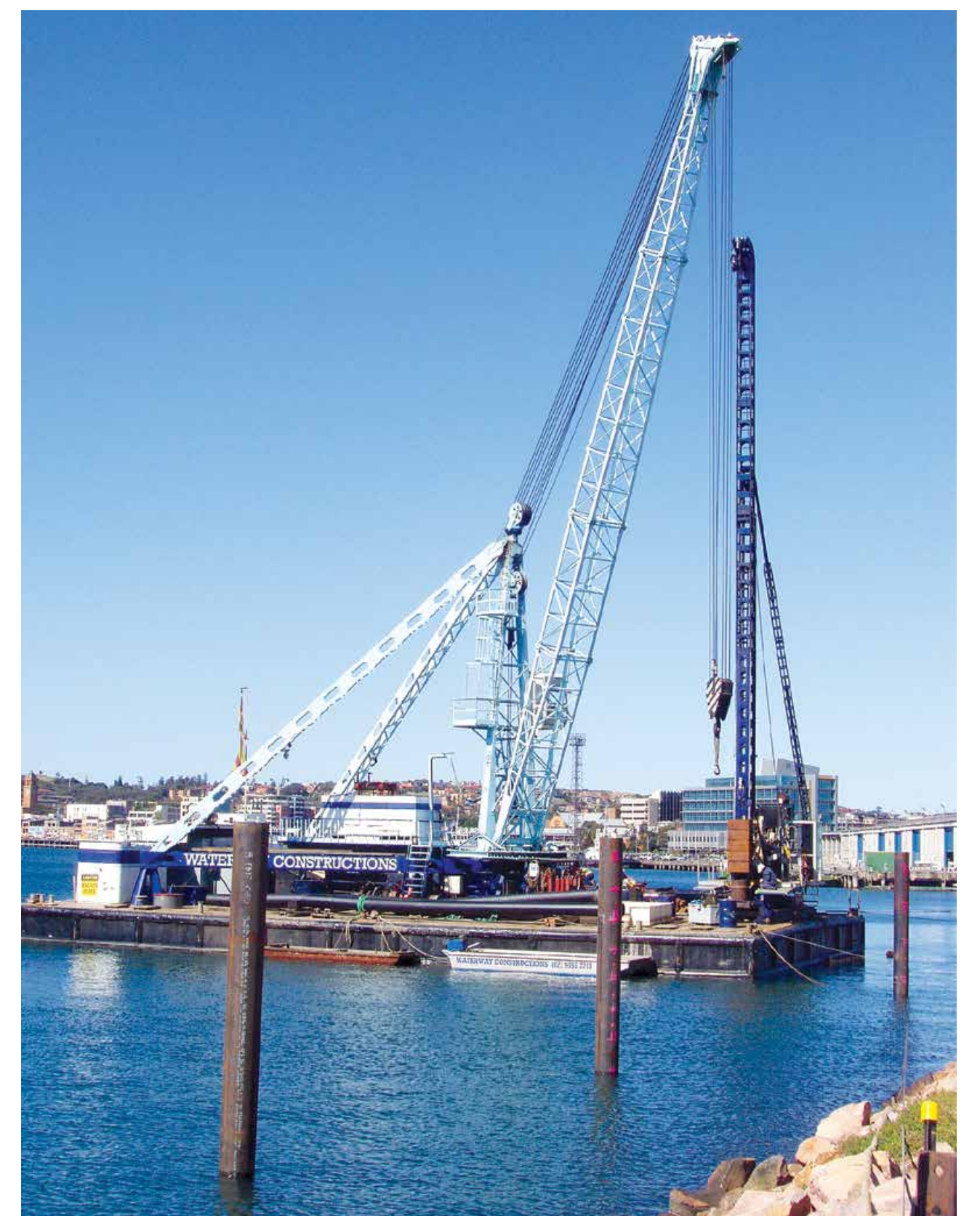
Barge-mounted cranes near a work site in Sydney Harbour
