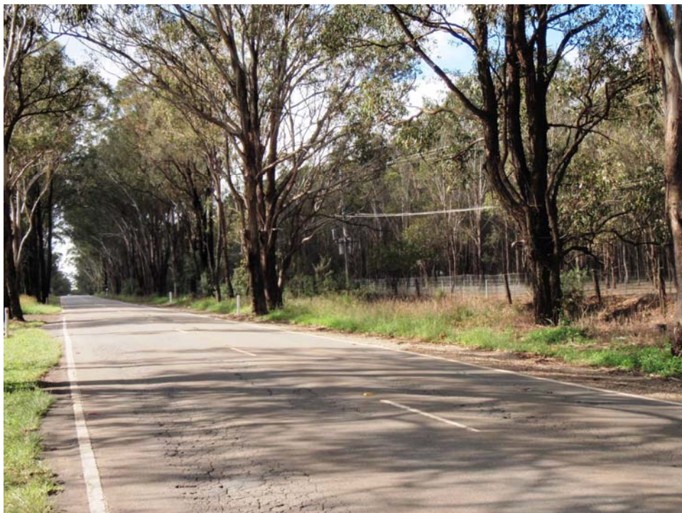
Existing Bringelly Road at Rossmore, view to the east.
