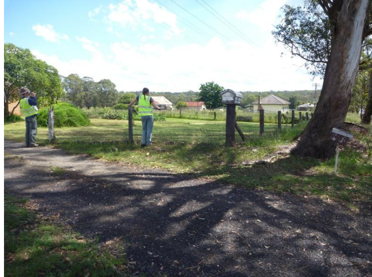
Plate 17. Driveway entrance with imported road base [REDACTED]
