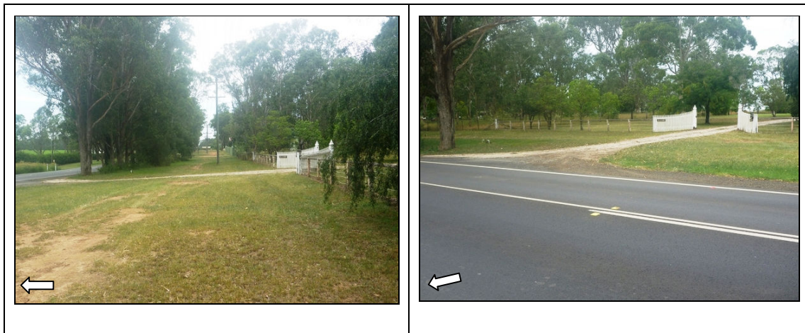
Figure 4.2: The LEP heritage listed house known as Allenby, 661 Bringelly Road, Rossmore (Lot 2 DP 546020). Both left and right photos show the proximity of Bringelly Road to the entrance gates and picket fence of the property. Source Austral Archaeology Pty Ltd DSCN 020, 021.
