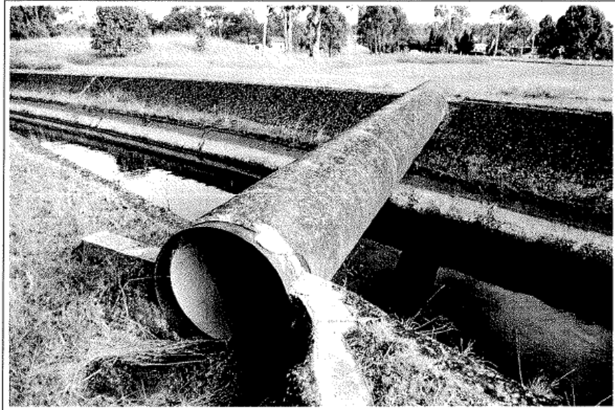
Caption Iron and concrete pipe flume.
