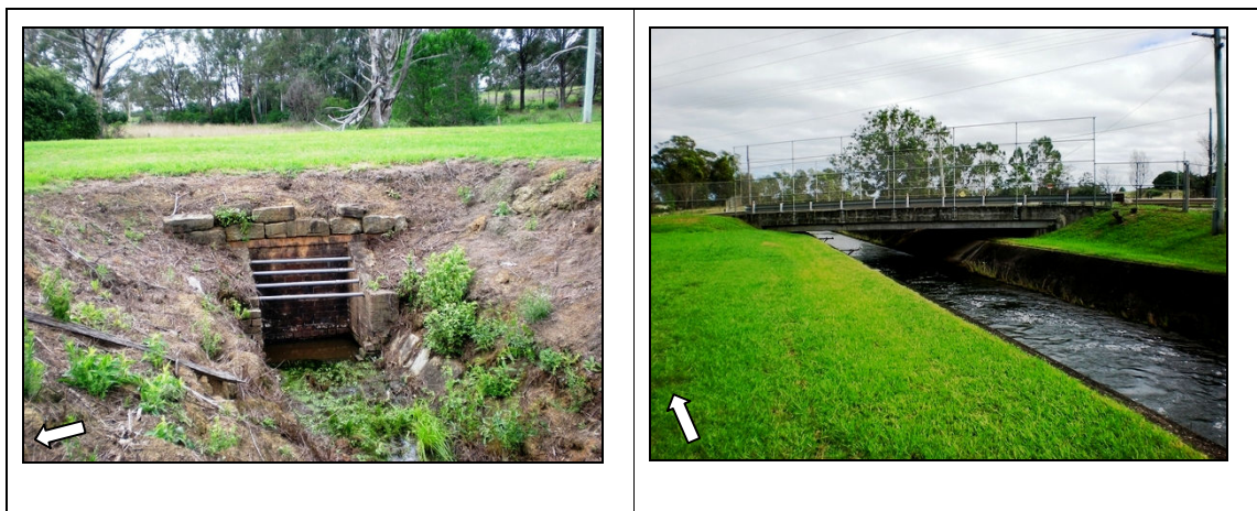
Figure 4.2: The Brick Culvert (CMP Item 28 – photo on the left) and Canal Overbridge located on Bringelly Road built c. 1950s to 1960s (CMP Item 33 – photo on the right). Both items are part of the State heritage listing for the Upper Canal that passes through the study area (Lot 1, DP 725231 on south side of Bringelly Road). White arrow indicates North. (Source Austral Archaeology Pty Ltd DSCN 2822, 2828).
