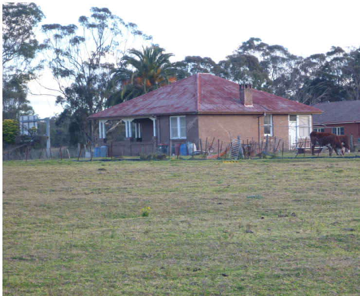
12 Bringelly Road, Horningsea Park (Lot 9 DP 29104). Cowpasture Rd frontage viewed to the southeast. Source Austral Archaeology Pty Ltd DSCN 220710040.
