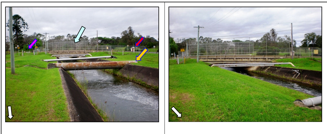
Figure 4.14: The photo on the left is a view to the south and shows several of the recorded items such as the flumes located within the Upper Canal that passes through the study area that includes CMP Item 35 (indicated by orange arrow); the Canal Overbridge located on Bringelly Road CMP Item 33 (indicated by blue arrow) and also shown in the photo to the right. Note former worker's cottage outside toilet in the background (indicated by red arrow) and location of access road gate CMP Item 34 (indicated by pink arrow) and also shown in Figure 4.15. White arrow indicates North. (Source Austral Archaeology Pty Ltd DSCN 2835, 2836).
