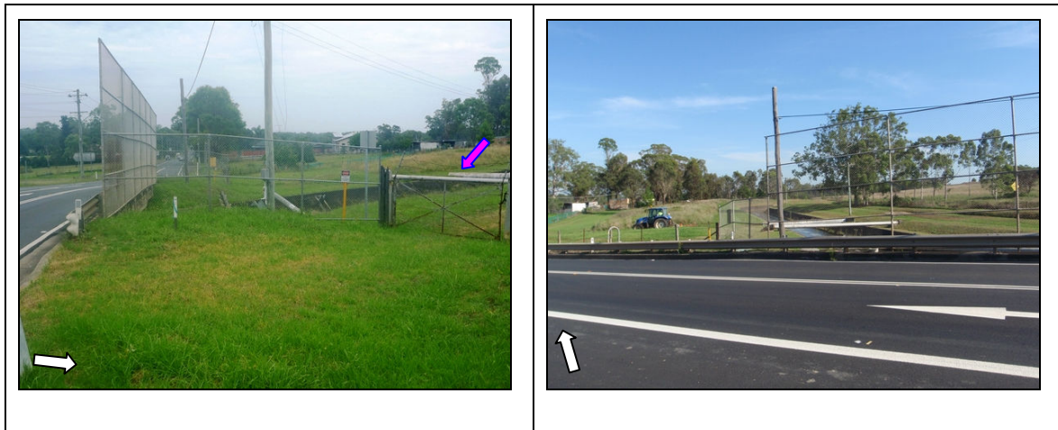
Figure 7.19: The photo on the left shows the Canal Overbridge (CMP Item 33) and associated fencing crossing over the Upper Canal in relation to the current alignment of Bringelly Road (view to the west). Note also the access road gate (CMP Item 34) located to the north (indicated by pink arrow). The photo to the right is the view to the north of the Canal Overbridge (CMP Item 33) in relation to the current alignment of Bringelly Road. White arrow indicates North. (Source Austral Archaeology Pty Ltd DSCN 038, P2110874).
