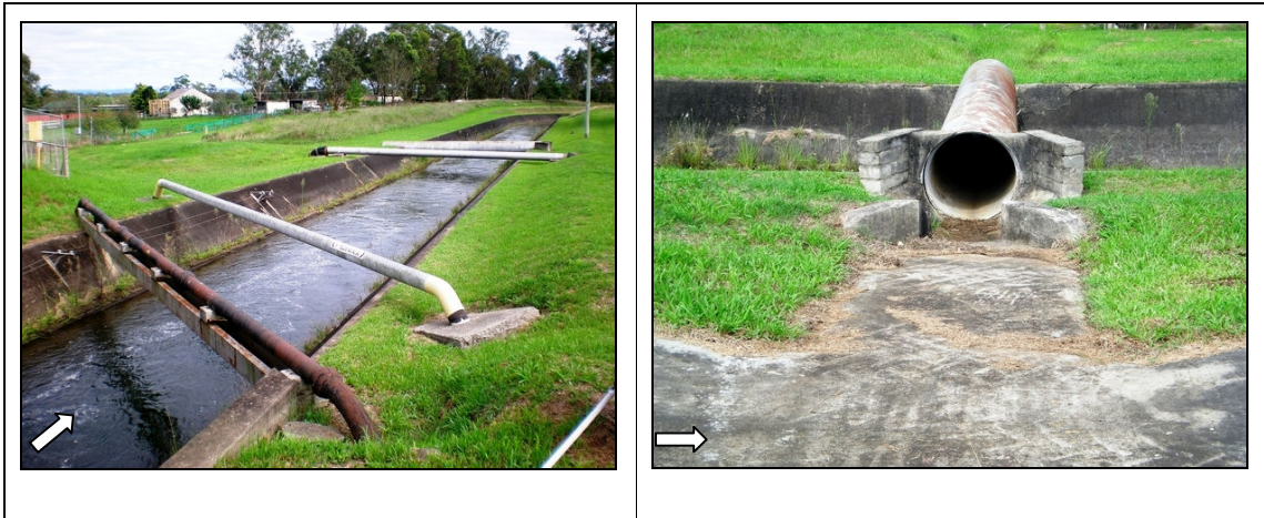
Figure 4.13: Photo on the left is a view to the west and shows a number of flumes that form part of the Upper Canal infrastructure along the north side of Bringelly Road and the photo on the right is a view to the west that shows the steel and concrete pipe flume dated c. 1960s (recorded in CMP (2002) to be intrusive and out of keeping with construction along the Upper Canal) (CMP Item 35). White arrow indicates North. (Source Austral Archaeology Pty Ltd DSCN 2832, 2834).
