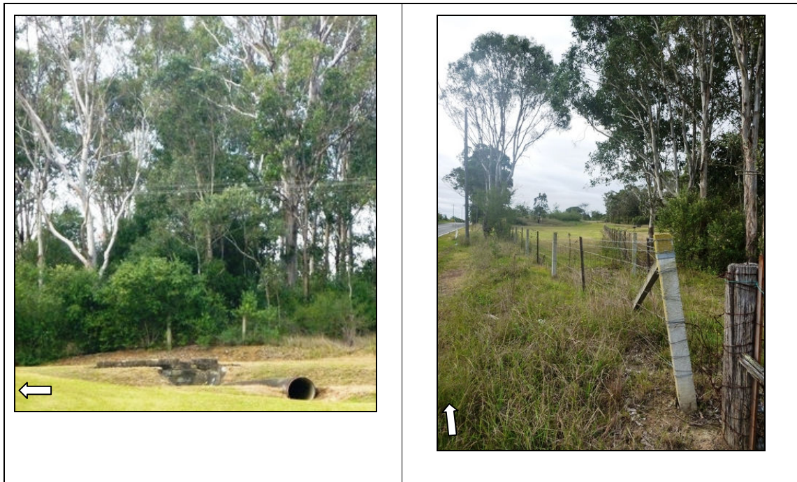
Figure 4.11: Photo on the left is a view to the east and is of the Iron and Concrete Pipe Flume (CMP Item 26) and the Stone Culvert (CMP Item 27) as well as fencing that relates to the former alignment of the Old Cowpasture Road which crossed the Upper Canal at this location. Photo on the right is a view to the north and shows the current fencing located at the intersection of the current alignment of Cowpasture Road and the previous alignment of Old Cowpasture Road (see also Figure 4.20). White arrow indicates North. (Source Austral Archaeology Pty Ltd DSCN 253, 259).
