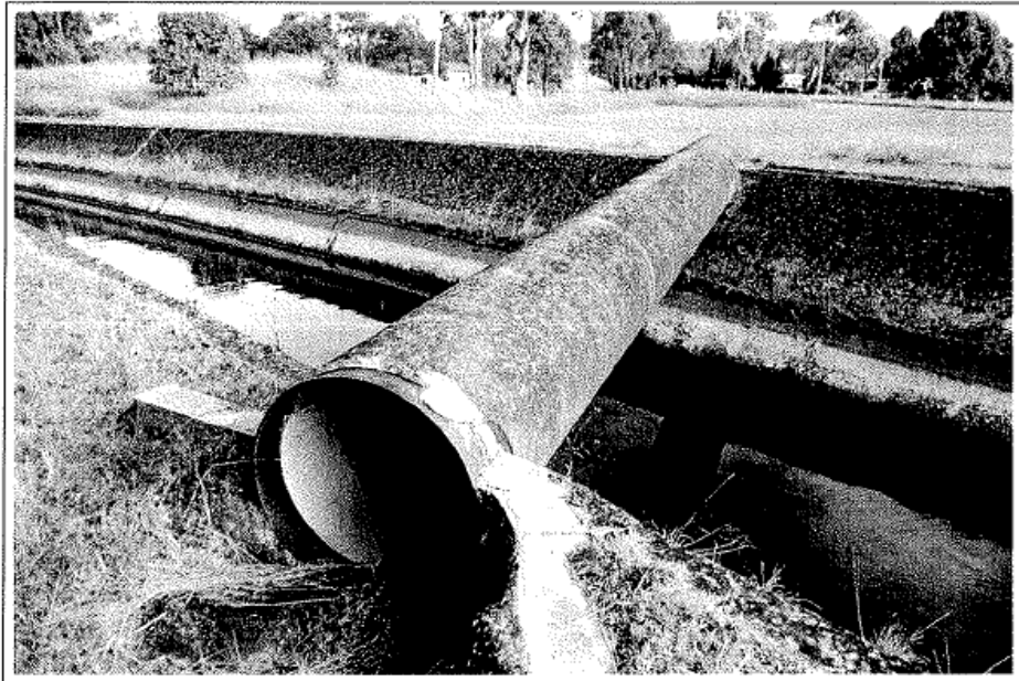
Caption Iron and concrete pipe flume.
