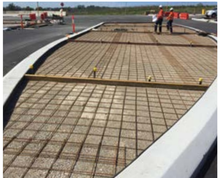
Building a concrete island on Skyline Crescent
