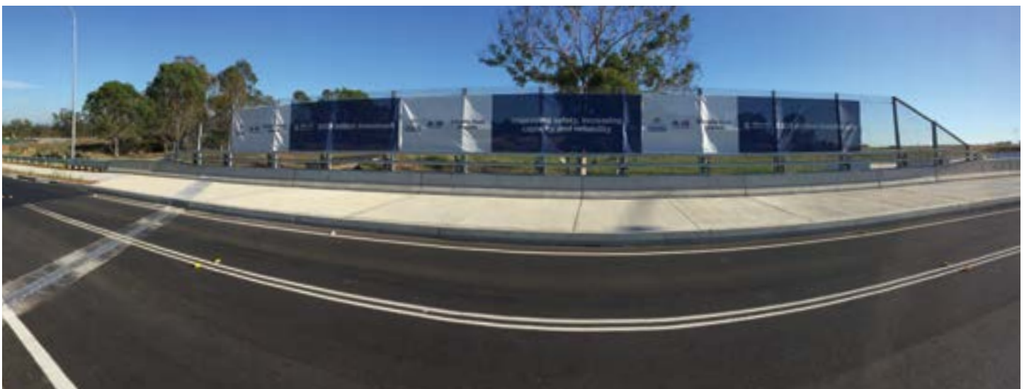
Upper Canal bridge on the newly built eastbound carriageway
