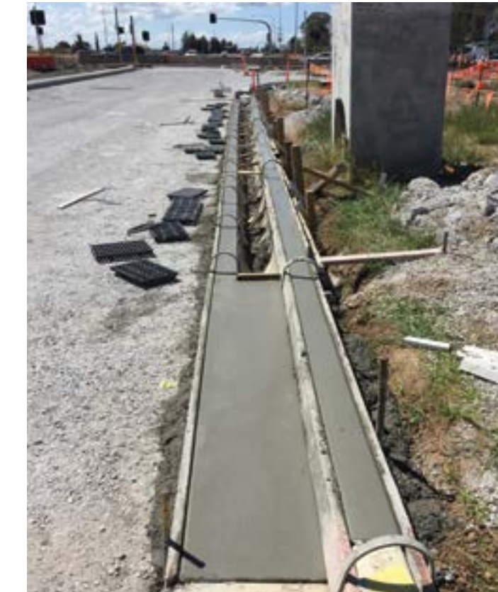
Building concrete drains on Bringelly Road, looking east near Camden Valley Way
